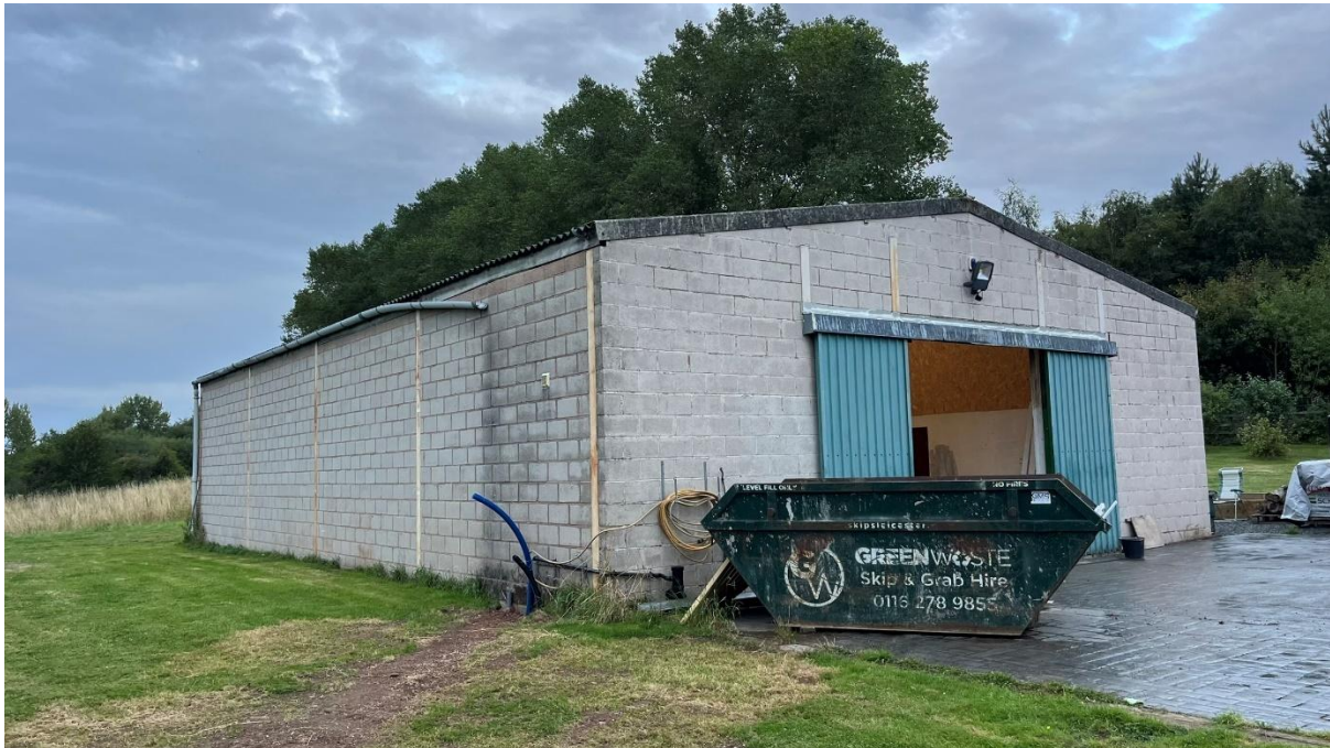
Photograph 1: The building taken from the south-west showing the breezeblock construction and large vehicle access doorway on the southern elevation.
