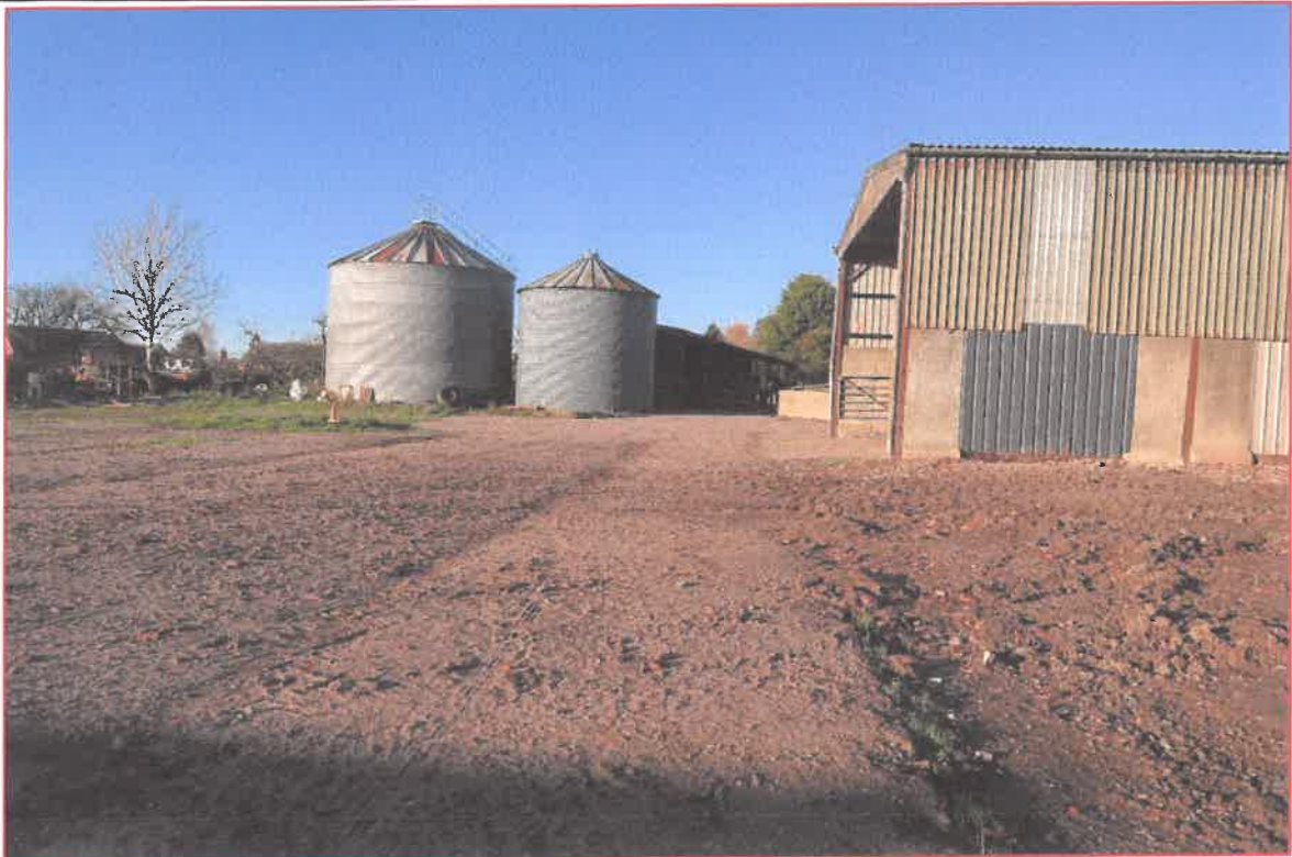
Fig. 2: View of existing
