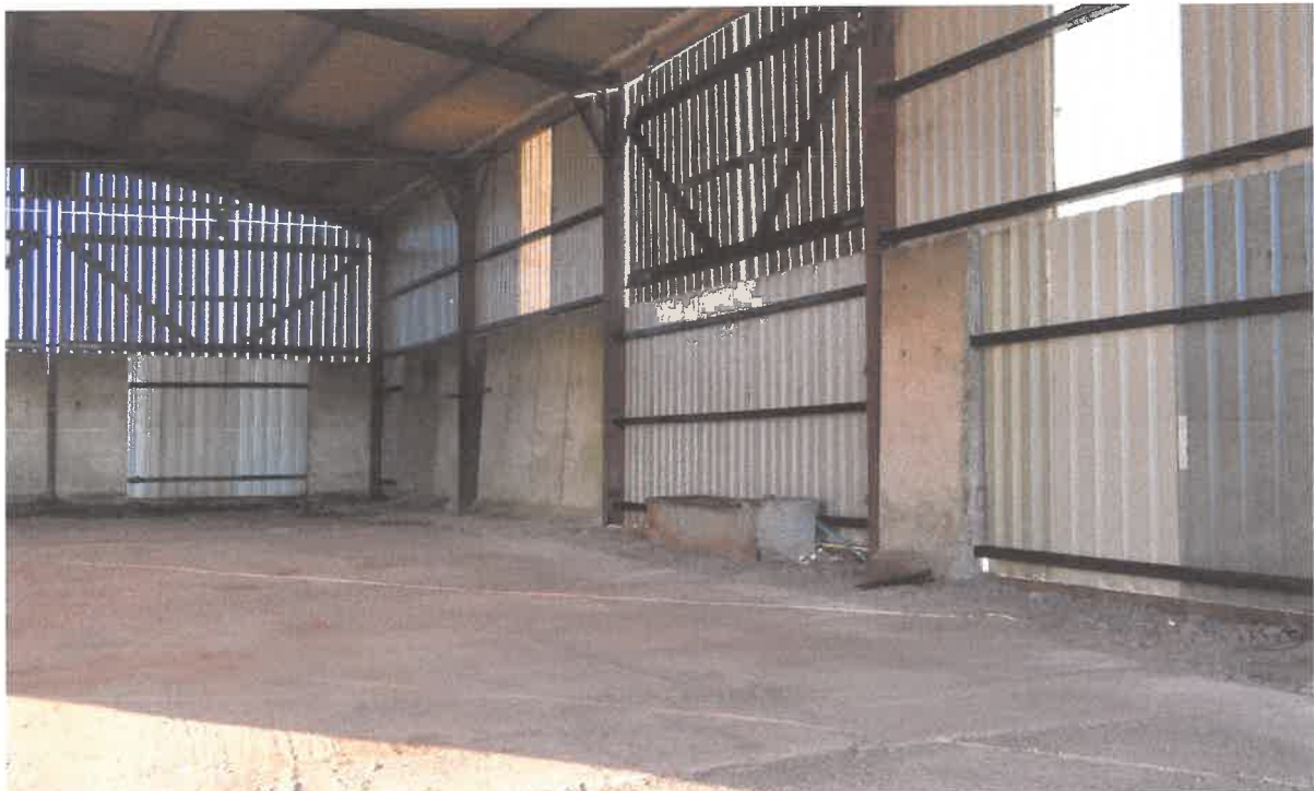
Fig. 3: View of existing
