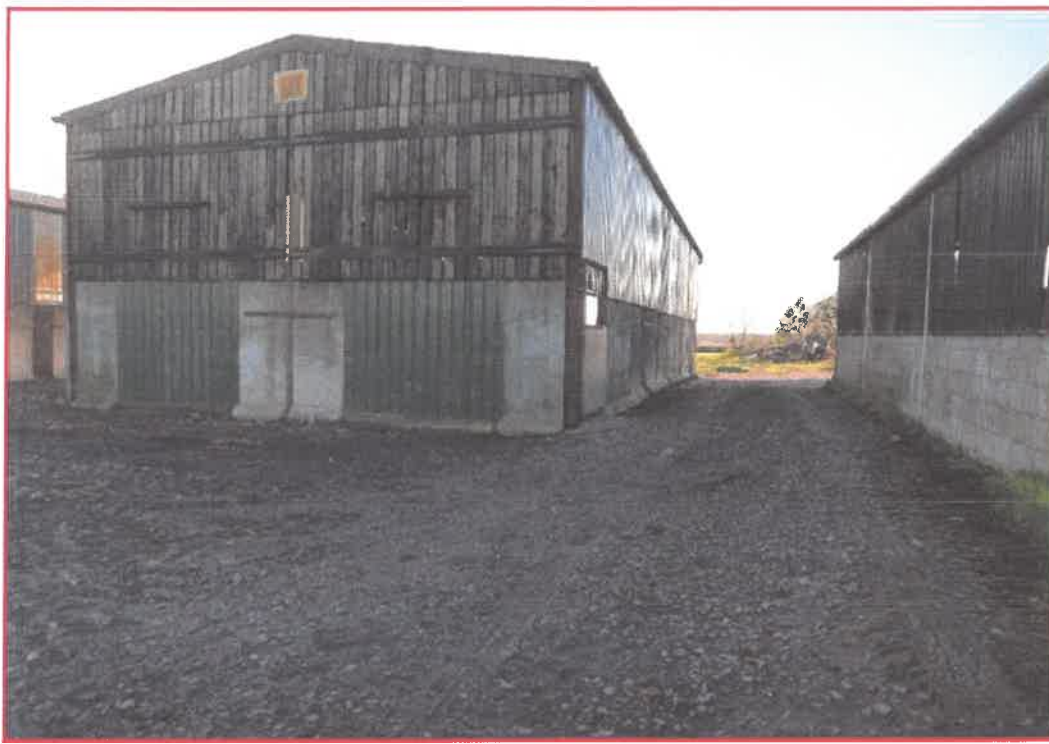
Fig. 4: View of site
