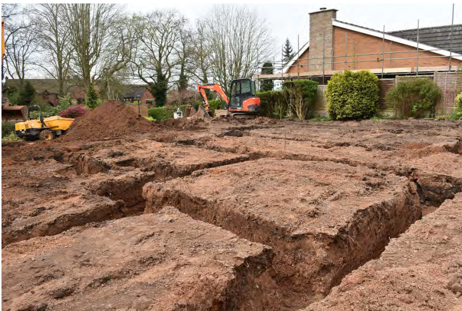
3 Excavated foundation trenches looking north-west
