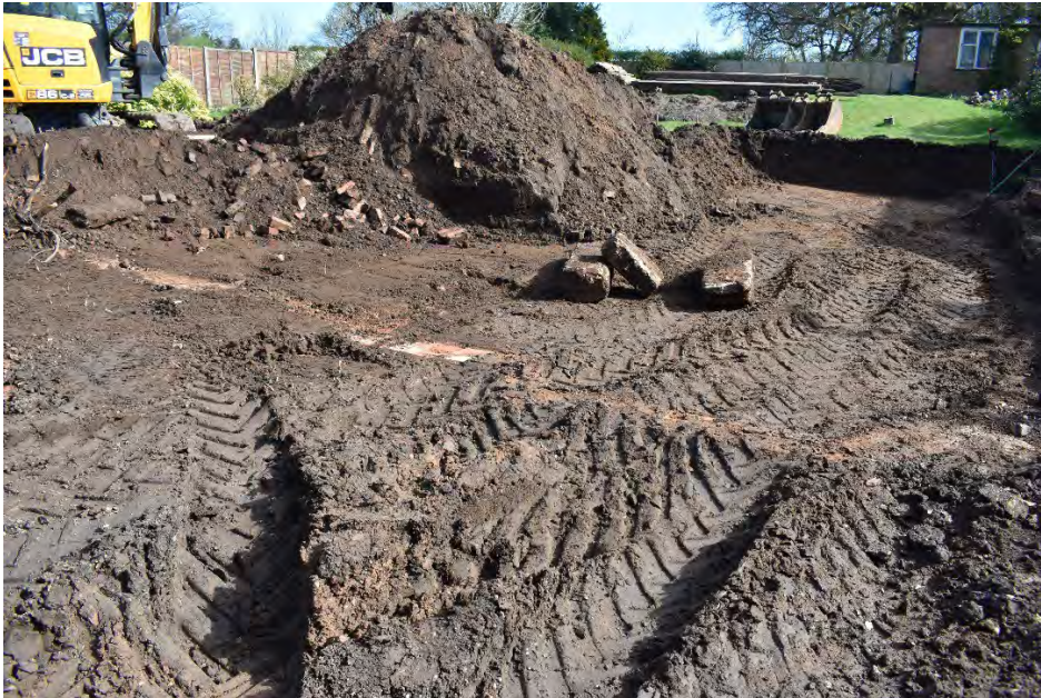
2 Working shot of ground reduction looking north-east
