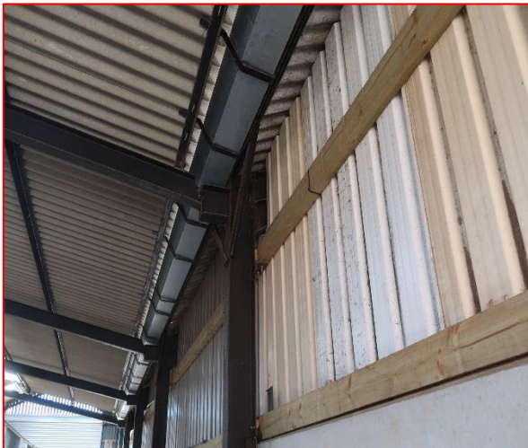
Internal view of Barn
