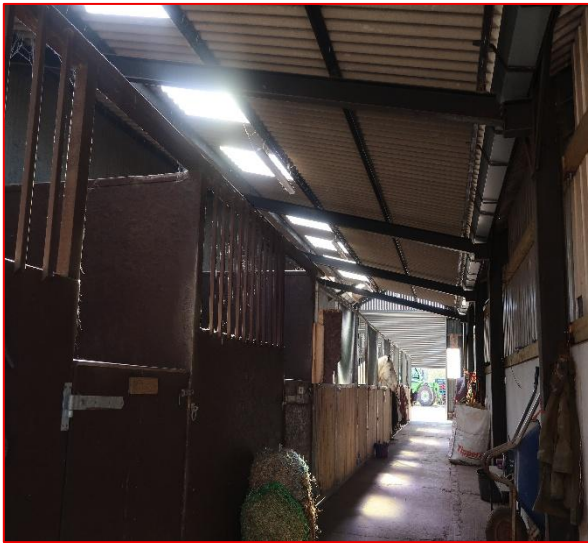
Internal view of Barn
