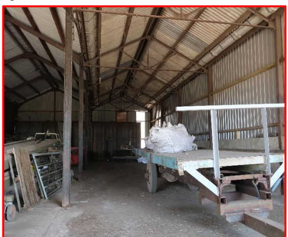
Internal view of Barn
