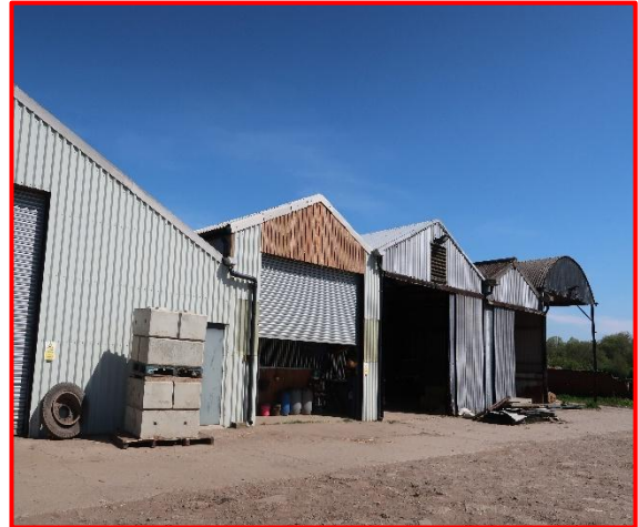
Fig. 2: – View of modern barns
