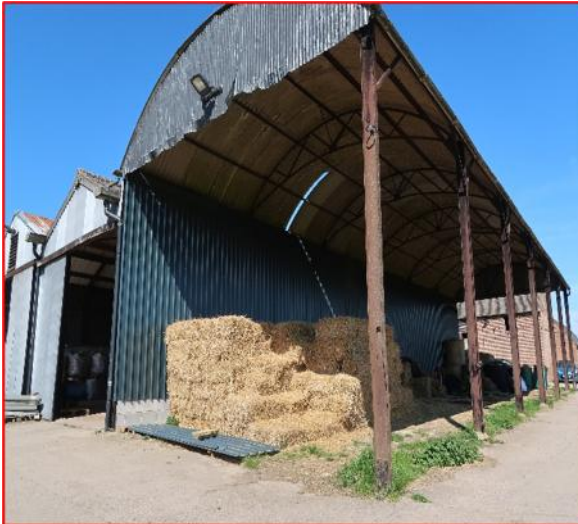
Fig. 3: – View of modern barns
