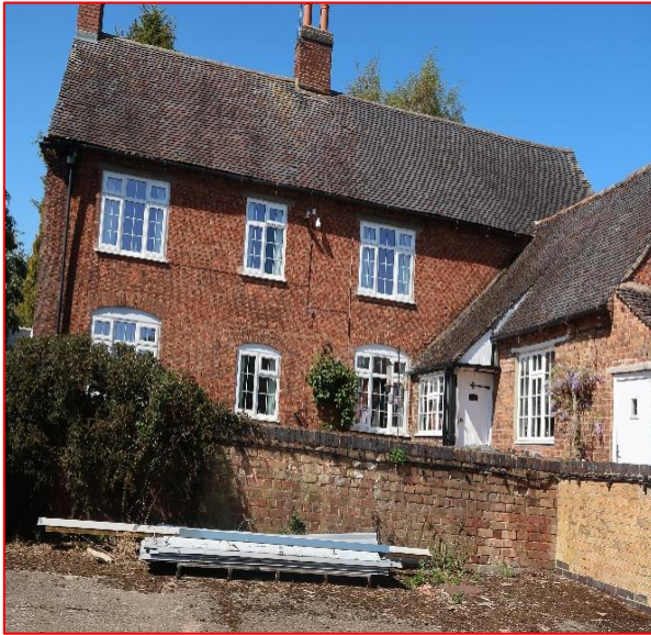
View of adjacent Farmhouse
