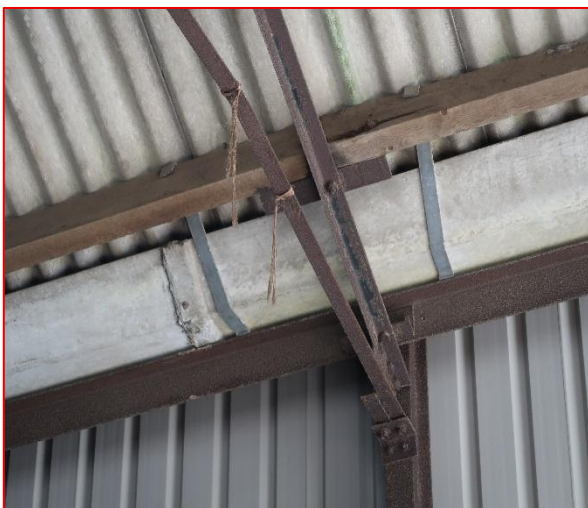
Internal view of Barn
