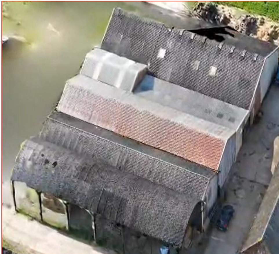
Fig. 1: view of site
