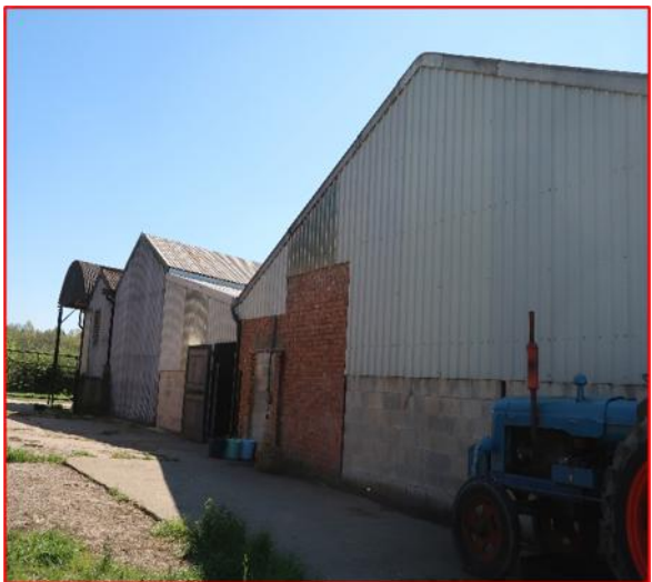
Fig. 4: – View of modern barns
