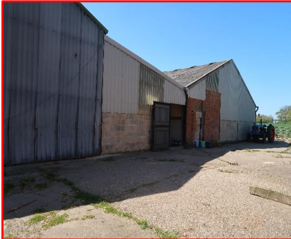
Fig. 1: – View of modern barns
