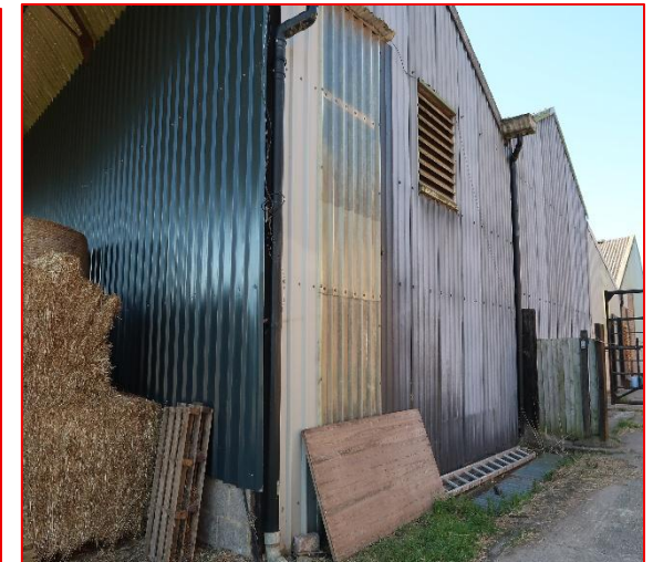
External view of Barns
