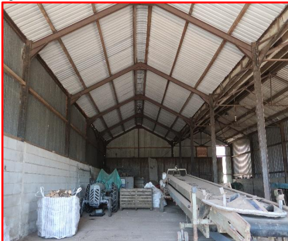
Internal view of Barn
