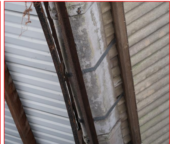
Internal view of Barn
