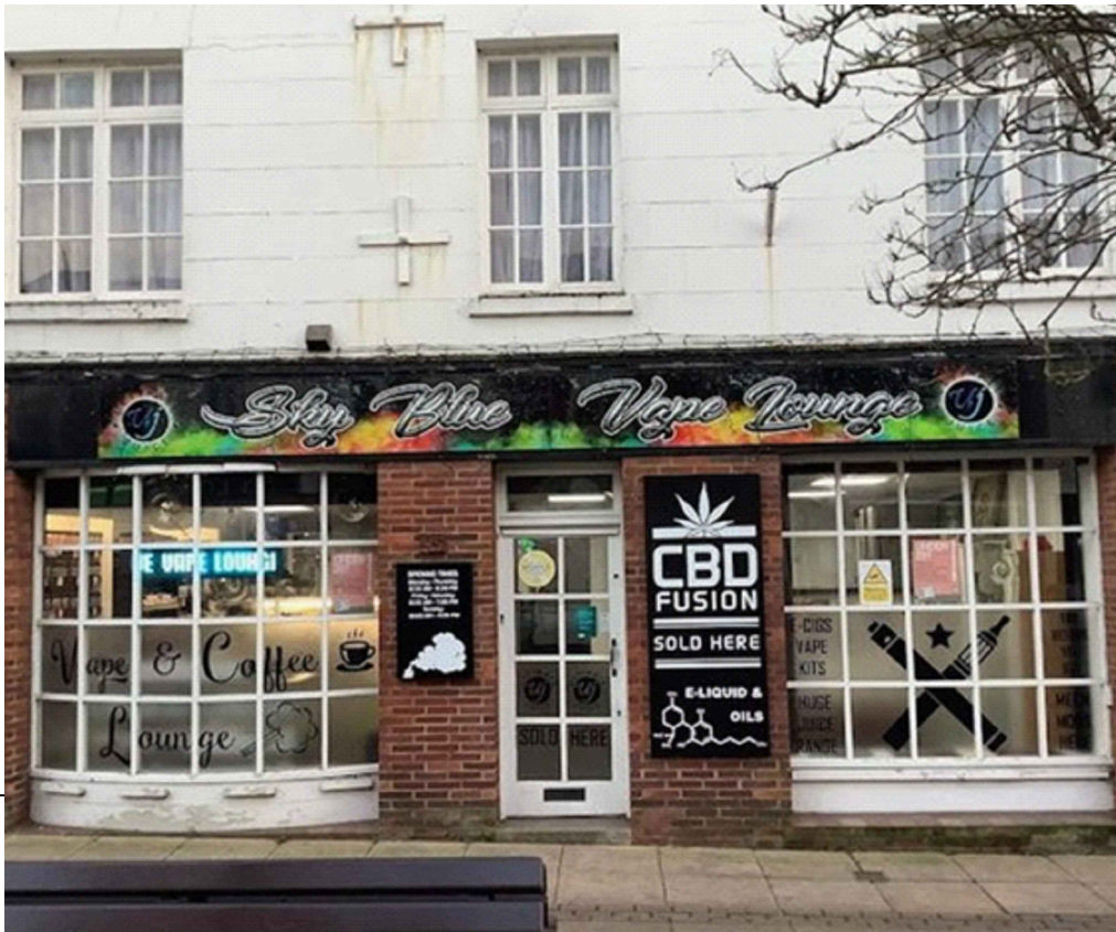
PREVIOUS FRONT VIEW
