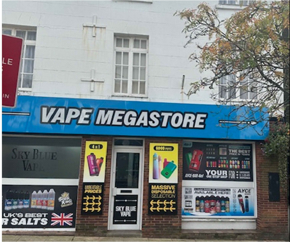
EXISTING FRONT VIEW
