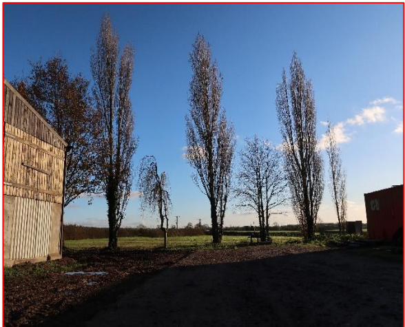
View of building & Poplar trees to boundary
