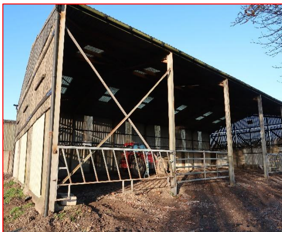
View of buildings.
