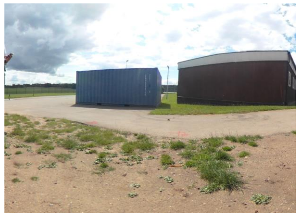
Photo 2 – Side view of 2no modular buildings
