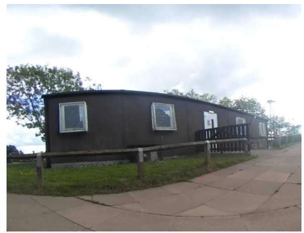
Photo 6 – Front view of modular building
