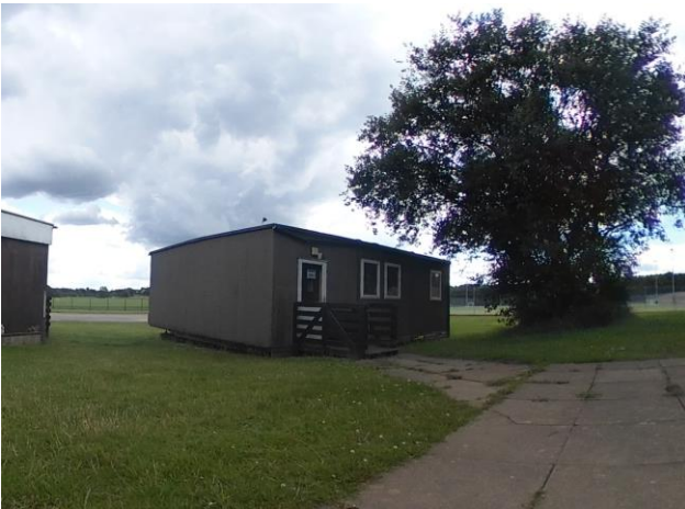
Photo 5 – Front view of modular building
