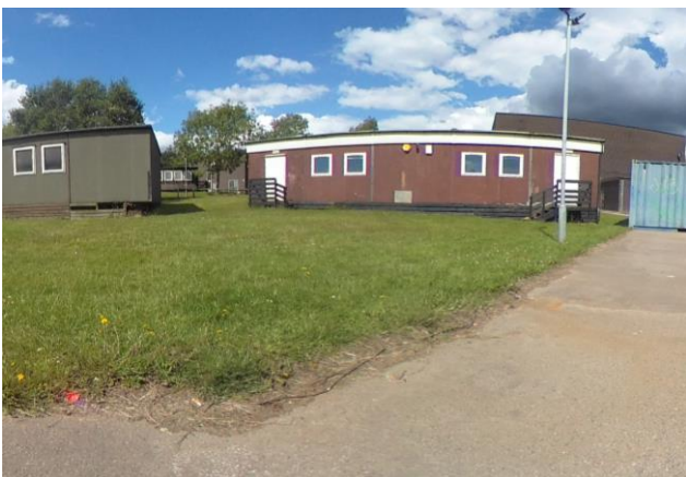
Photo 1 – Rear view of 2no modular buildings
