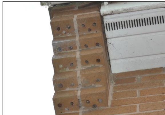
Photograph A1.4: Examples of missing mortar along some of the main gable verges.
