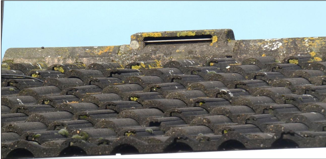
Photographs A1.2 (L) and A1.3 (R): The locations of the two narrow apertures at the ends of the soffit box below the eaves on the rear elevation are shown by the red arrows below left, and a close-up of one of these features is shown below right. There are similar apertures on the front elevation, however, those appear too narrow for bats to access.
