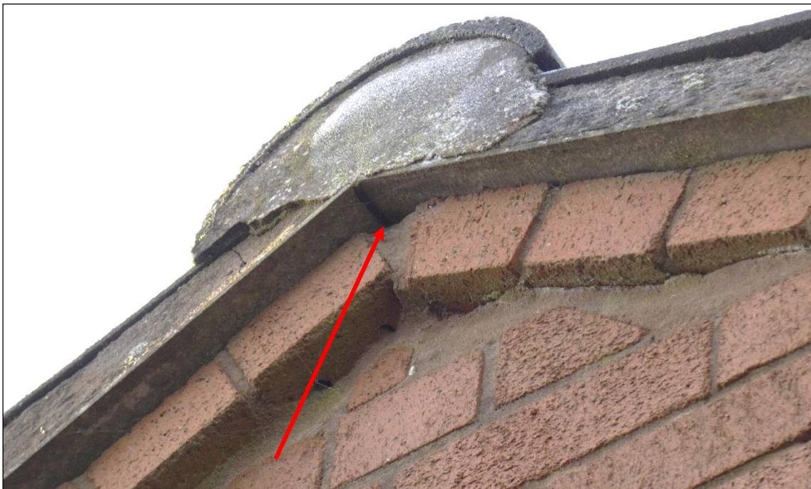
Photograph A1.7: The small aperture at the apex of the east gable wall (below the fibre cement lining).
