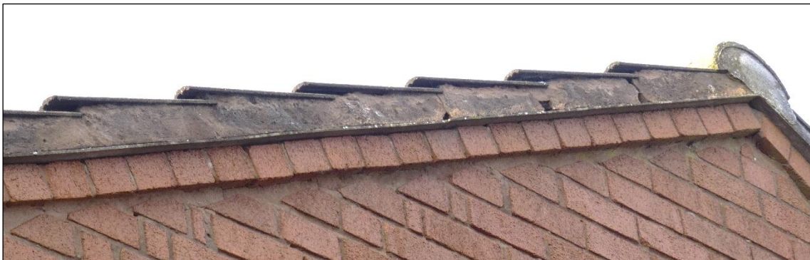
Photograph A1.4: Examples of missing mortar along some of the main gable verges.
