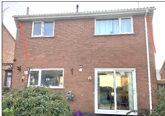
Photograph A1.4: Examples of missing mortar along some of the main gable verges.
