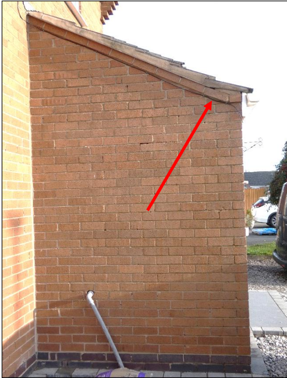
Photograph A1.7: The small aperture at the apex of the east gable wall (below the fibre cement lining).
