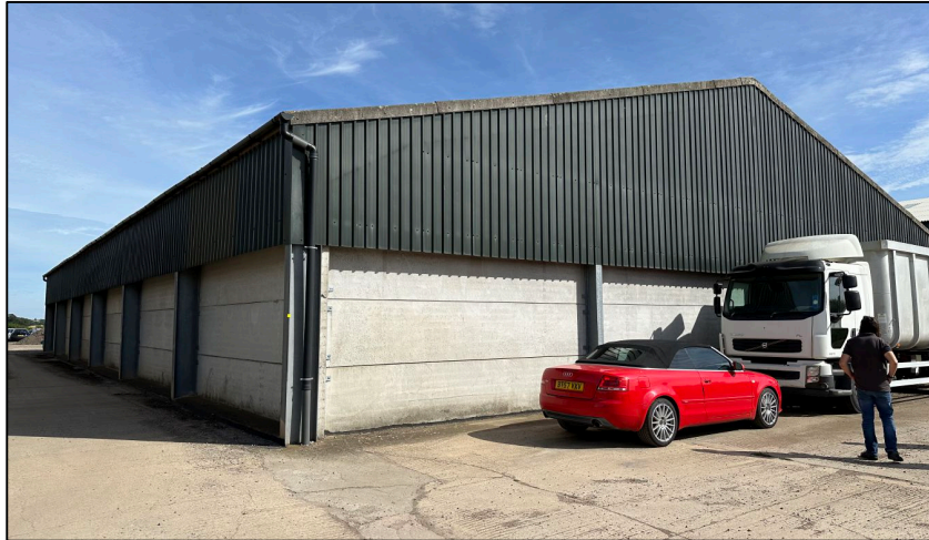
Photo 1. View of south and west elevations of proposed change of use building
