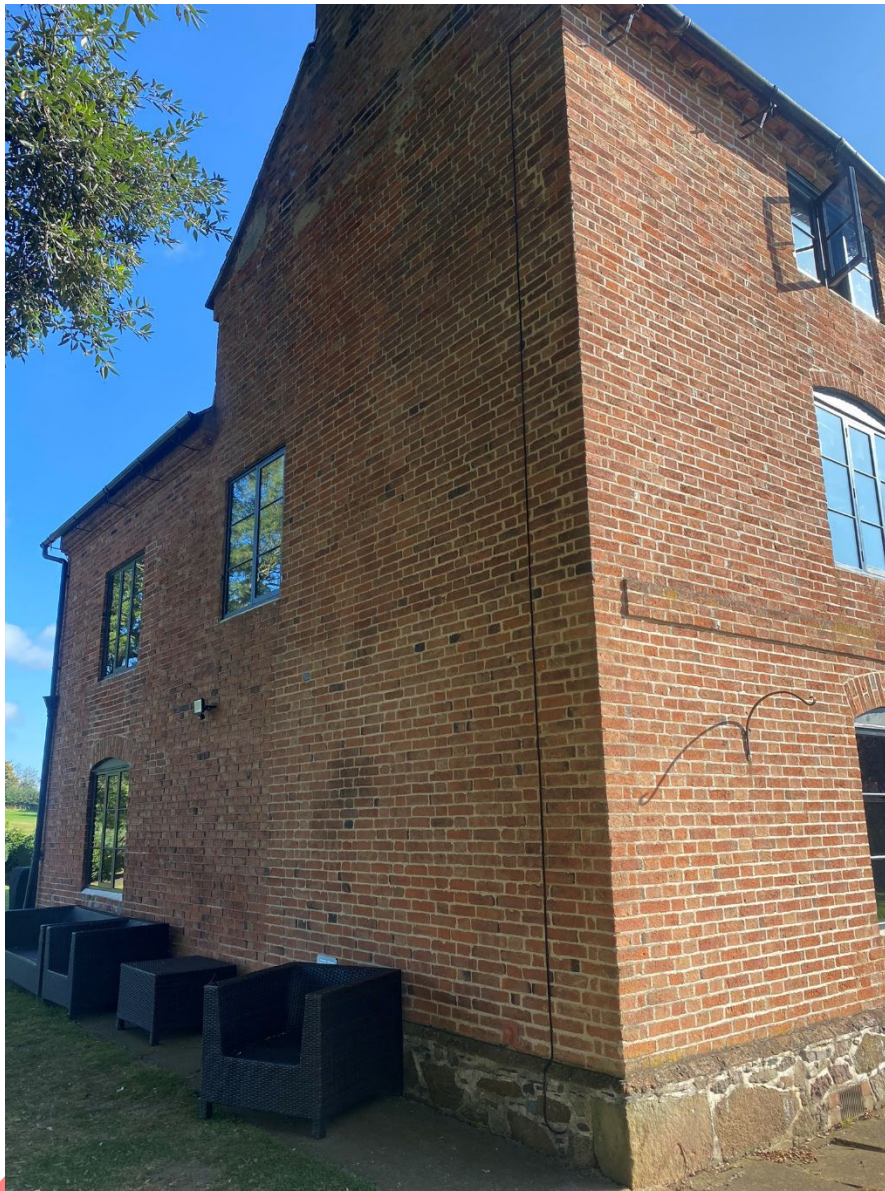
Figure 26: South-west corner of farm-house (Photo D)
