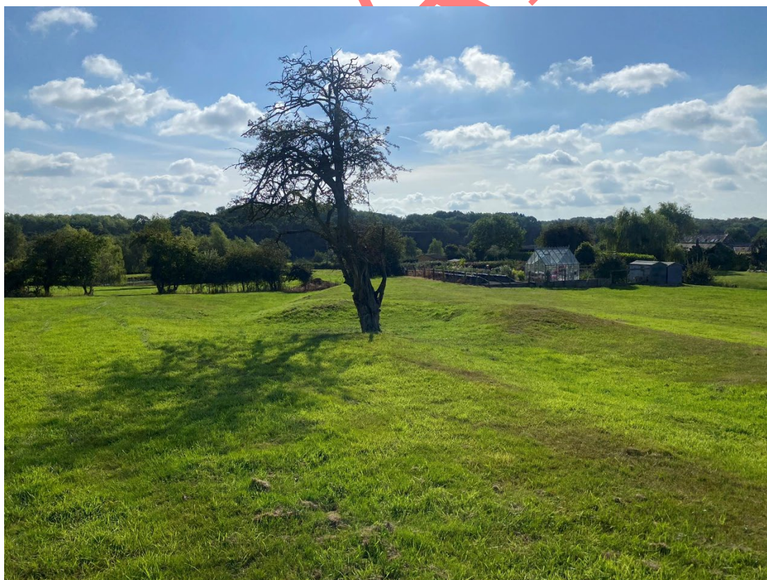
Figure 32: View of earthworks, looking east. (Photo J)
