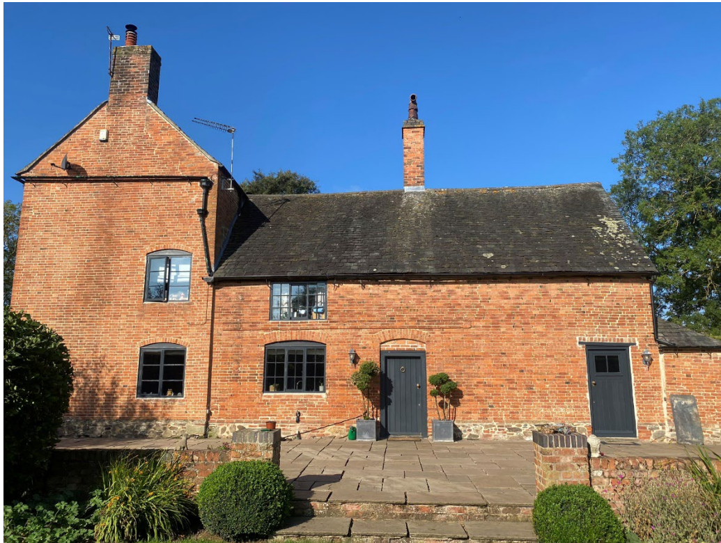
Figure 29: East facing wing of Old Hays Farmhouse. Likely the earliest part of the building, looking west. (Photo G)
