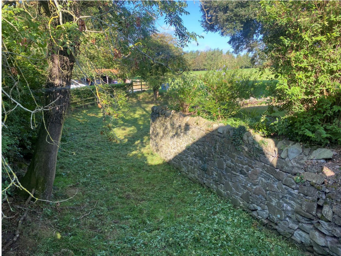
Figure 24: View of the moat from the bridge. Looking west. (Photo B)
