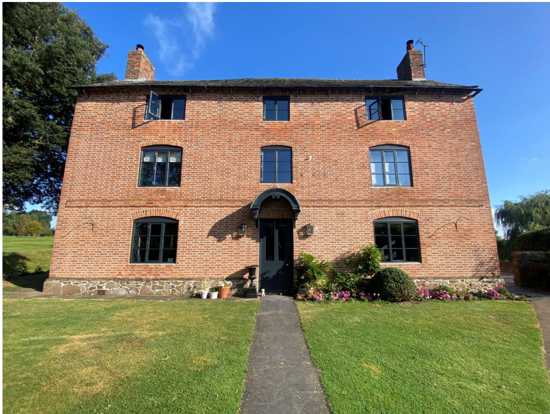
Figure 25: South face of Old Hays Farmhouse, looking north.
