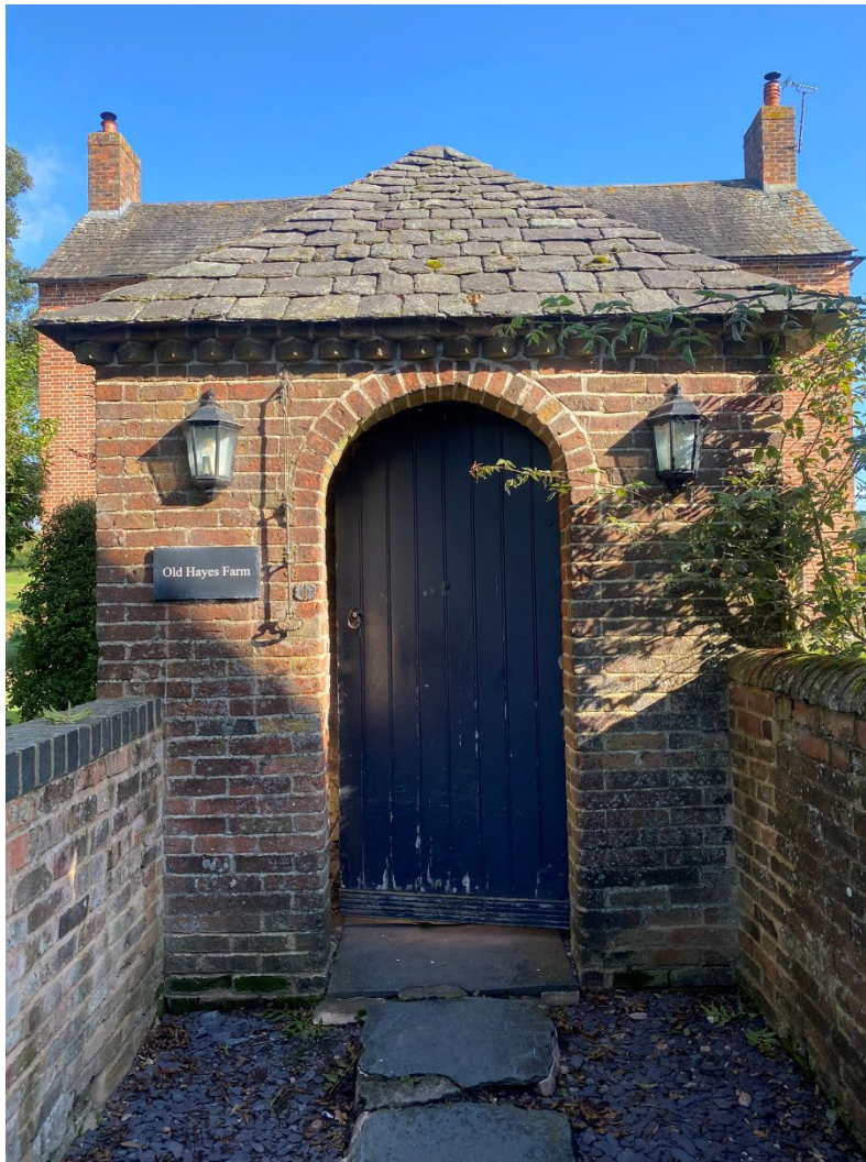
Figure 23: Photo A. Entrance to the gatehouse, looking north.
