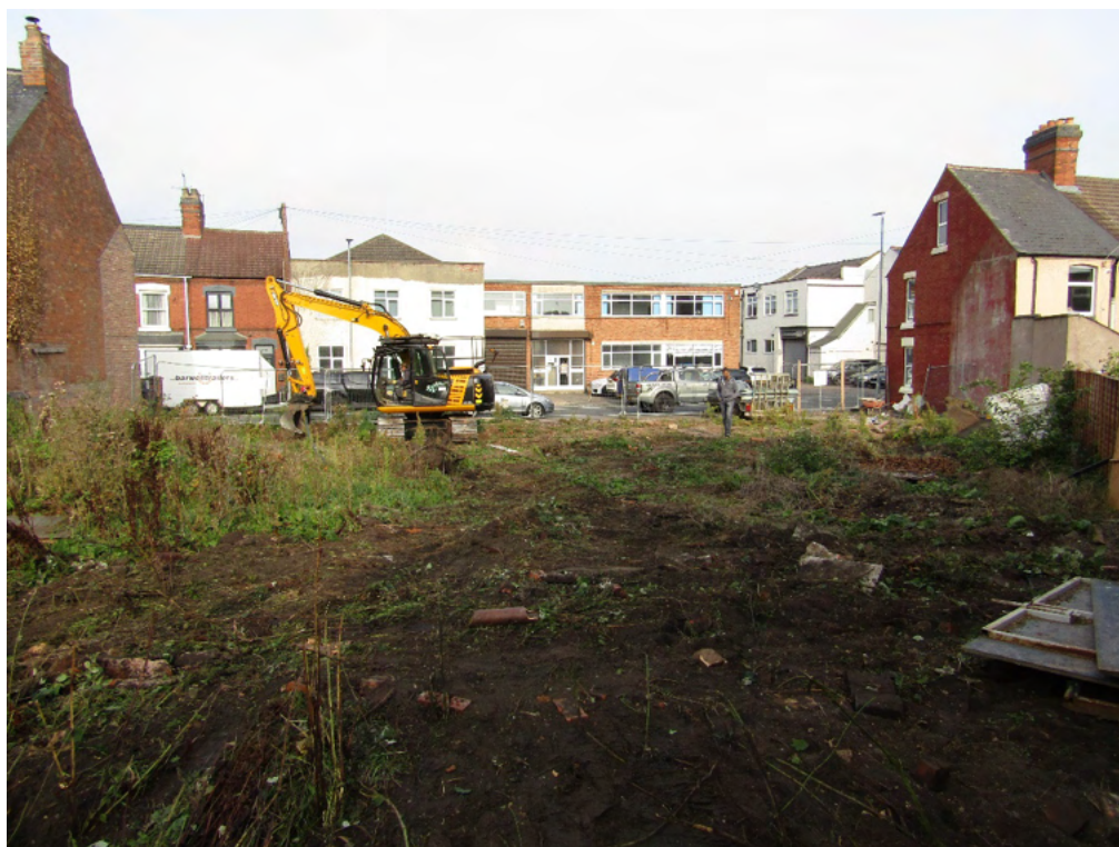
Figure 7: Area prior to stripping looking north-west.
