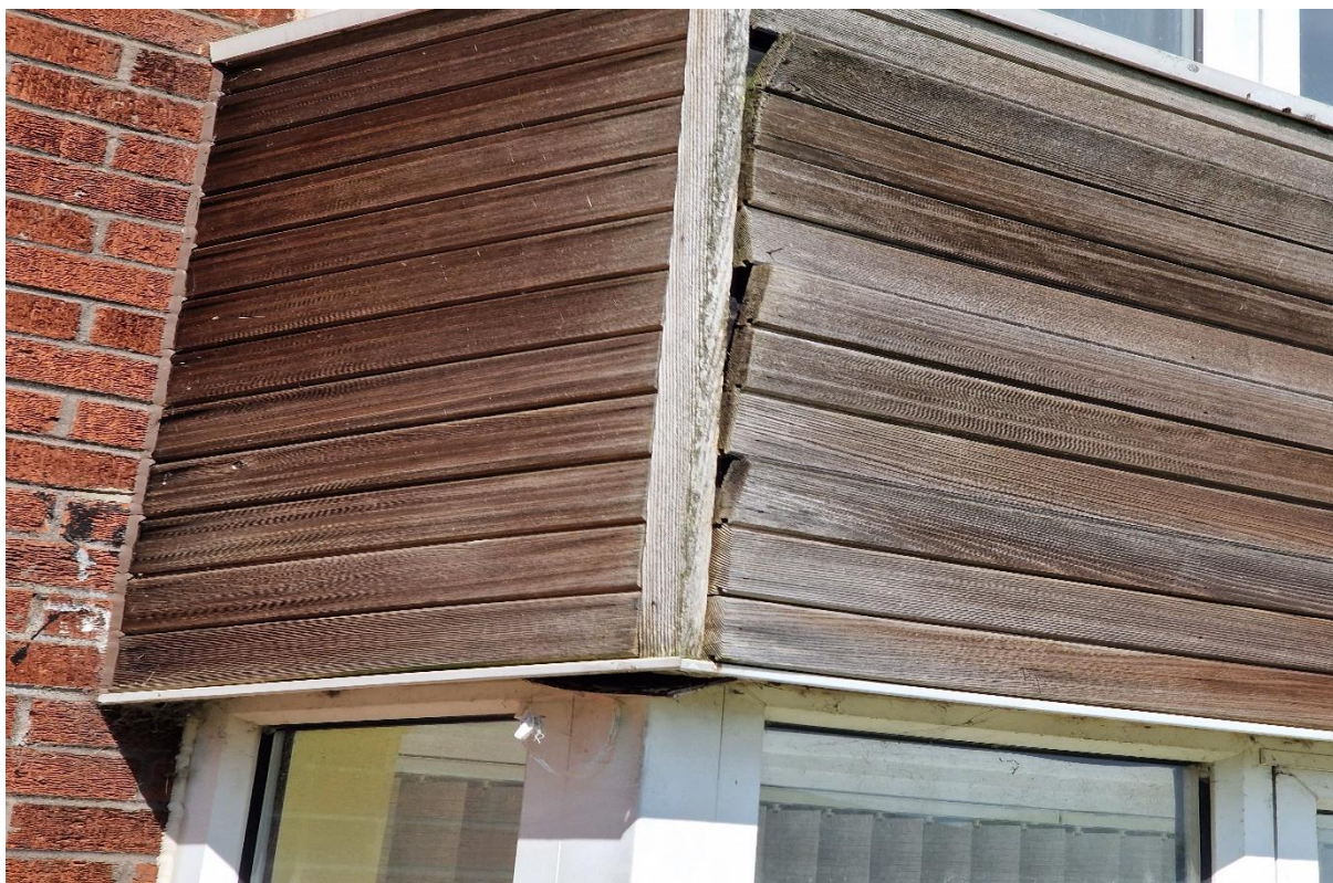
Plate 8: Image showing the missing wood panels on B3 .
