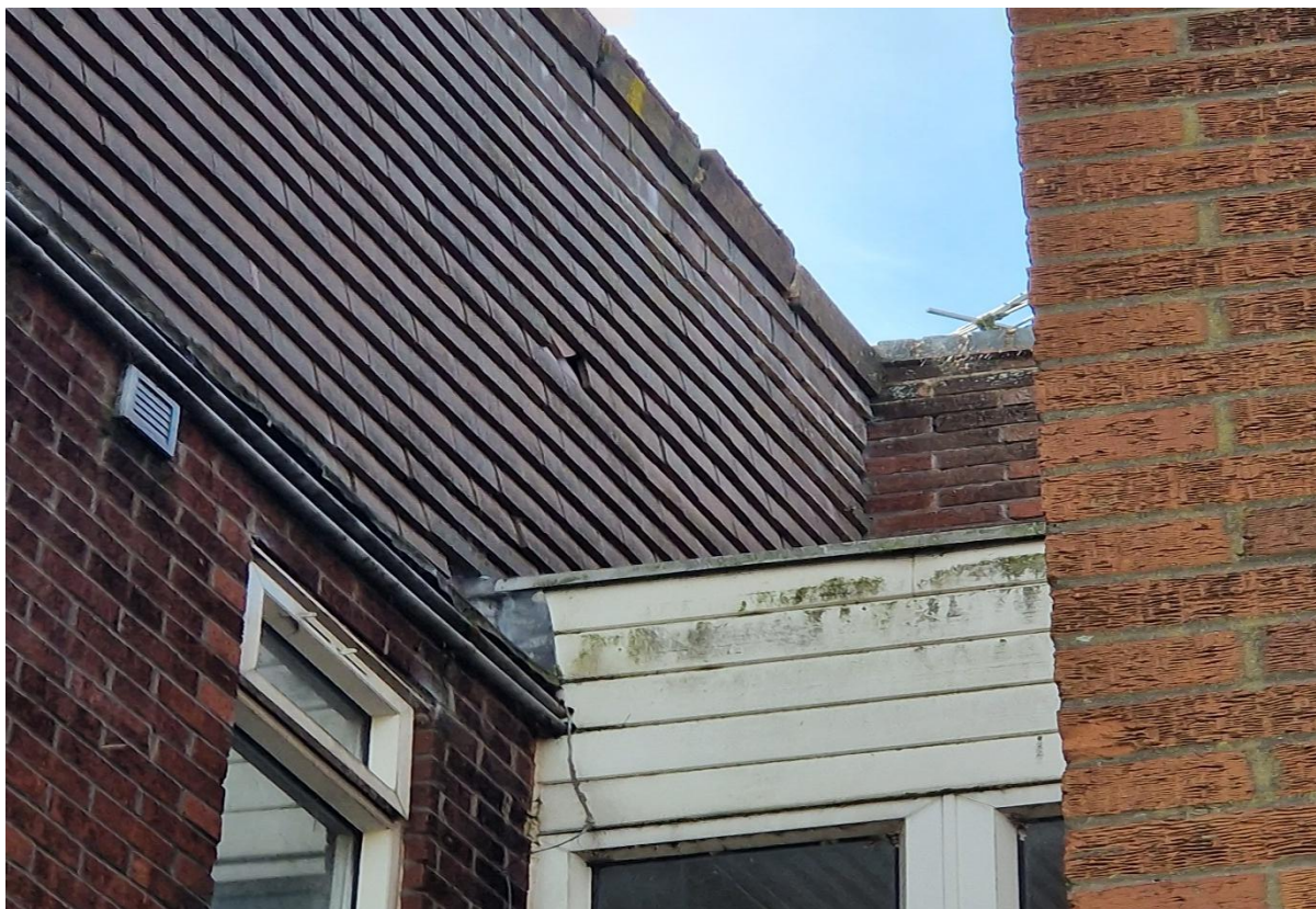
Plate 5: Image showing the missing edge tile on B1 .
