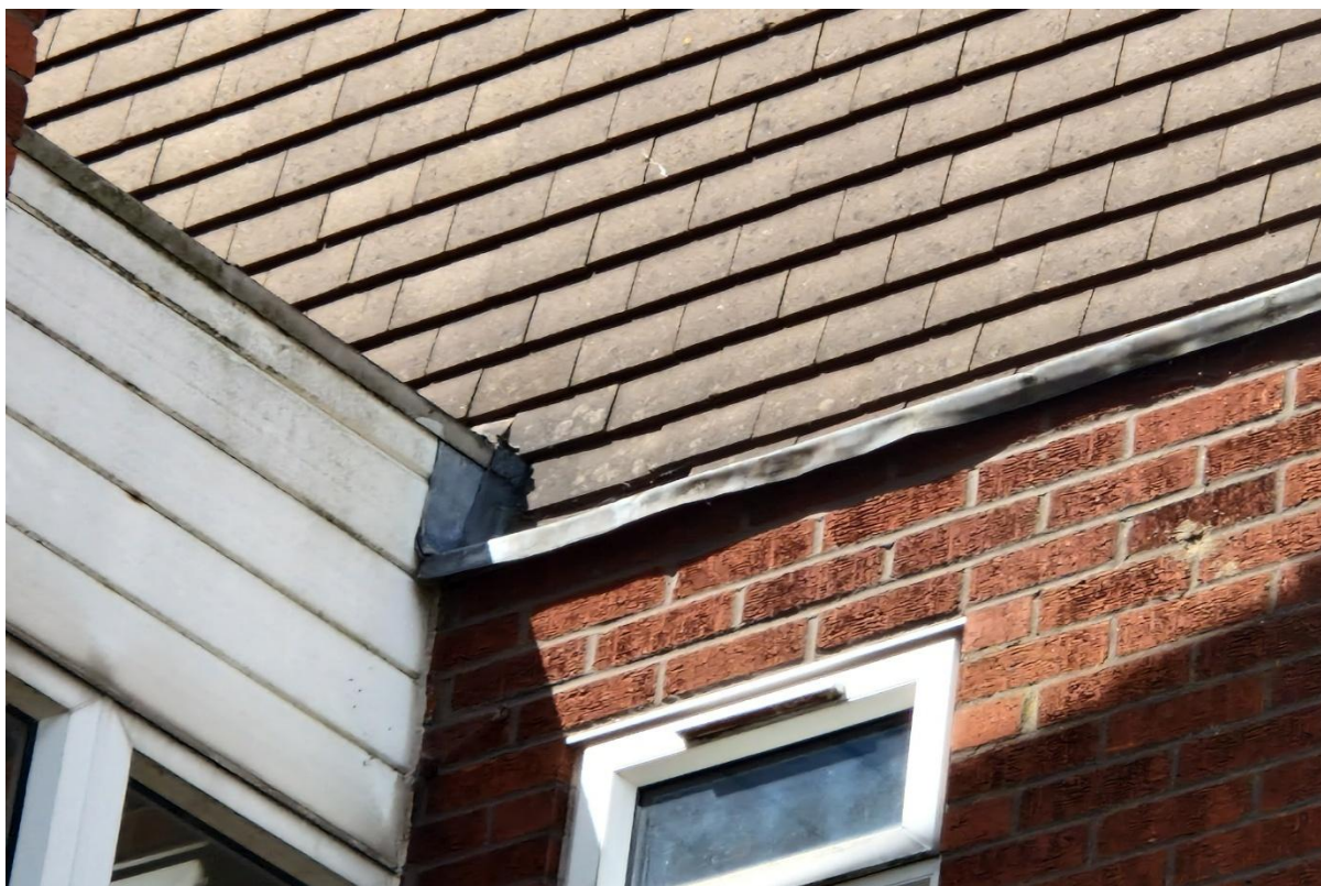
Plate 6: Image showing the vent in flashing part of B2 .
