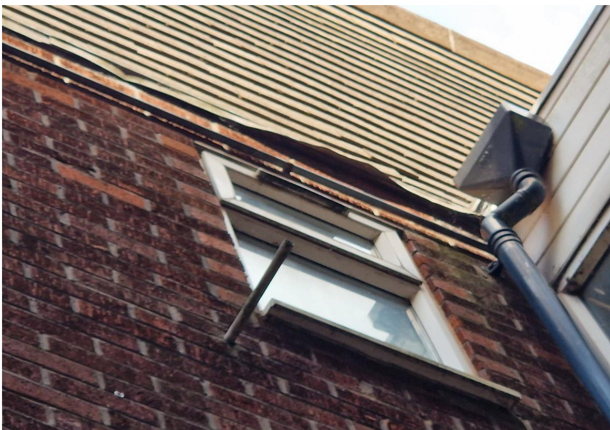
Plate 4: Image showing the lifted flashing on the southern elevation of B1 .
