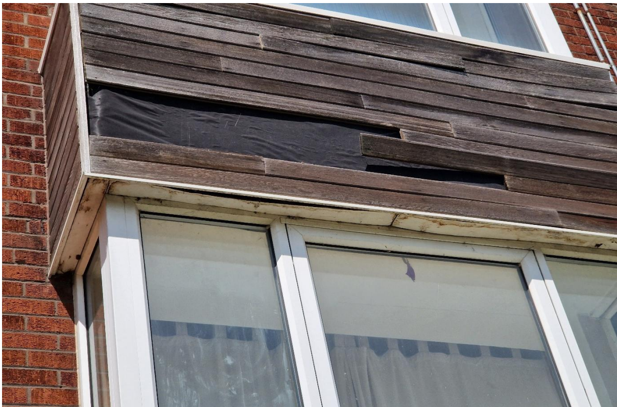
Plate 2: An image showing the missing wood panels on B3 .
