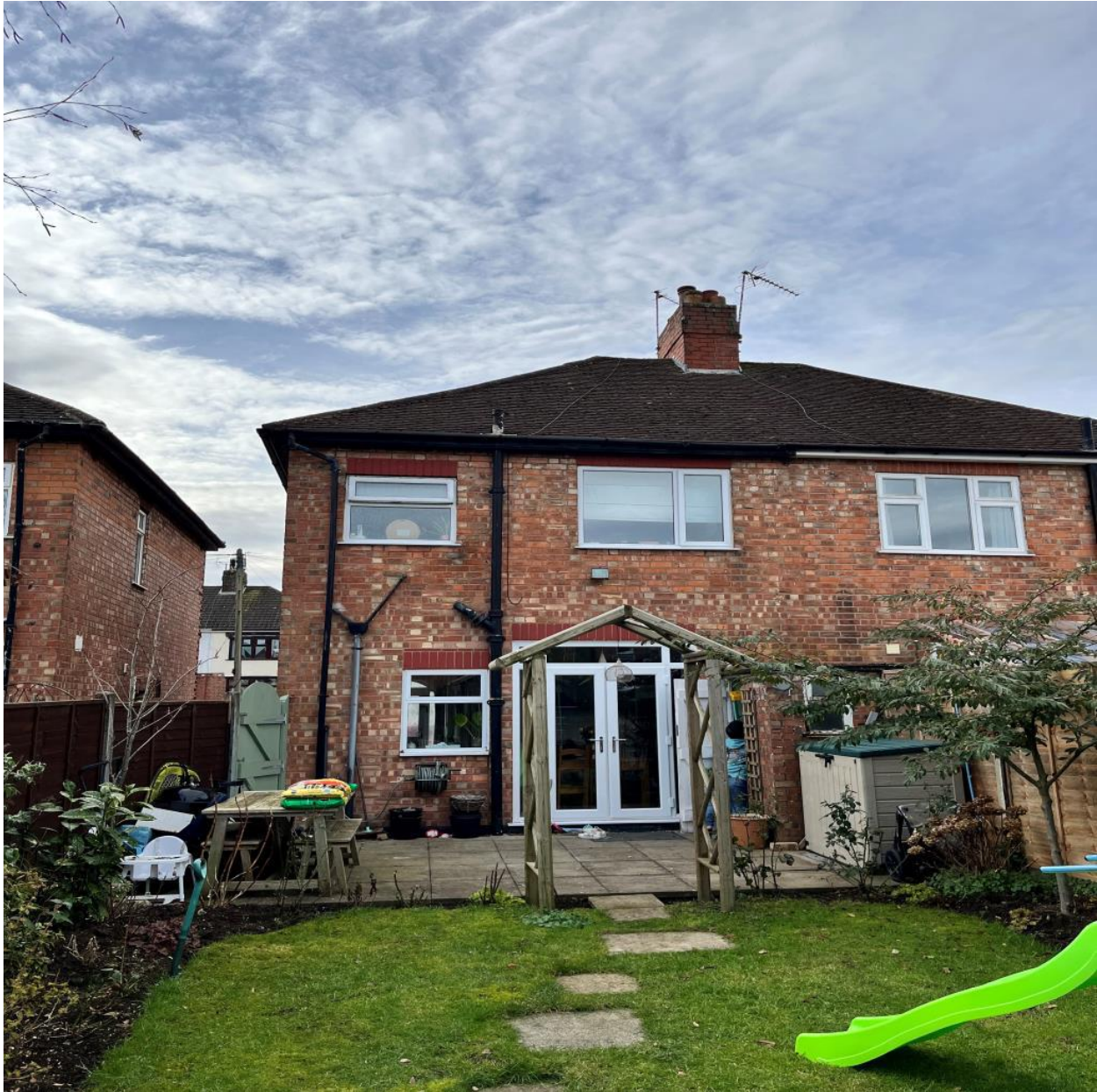
Photograph 2. The Rear Elevation
