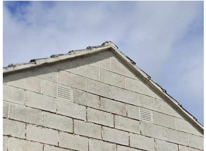
Sealed eaves of eastern building
