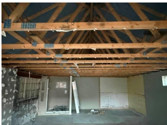
Upper floor of eastern building
