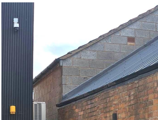
North and east elevations of eastern building
