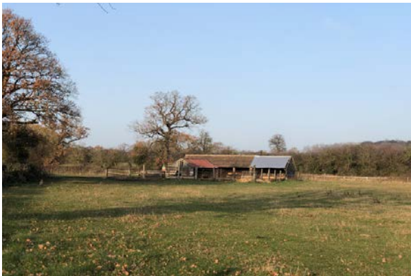
Barn buildings viewed from south
