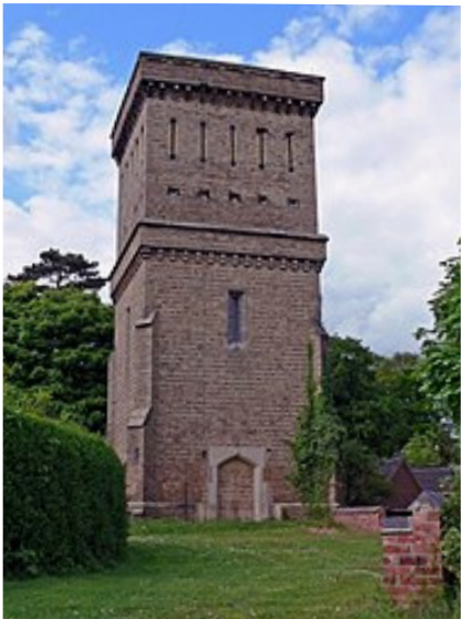
Ashby Water Tower
