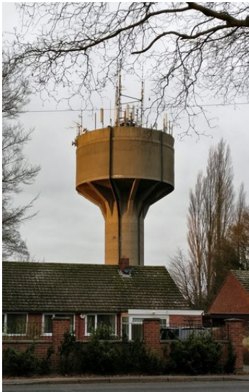
Barwell Water Tower
