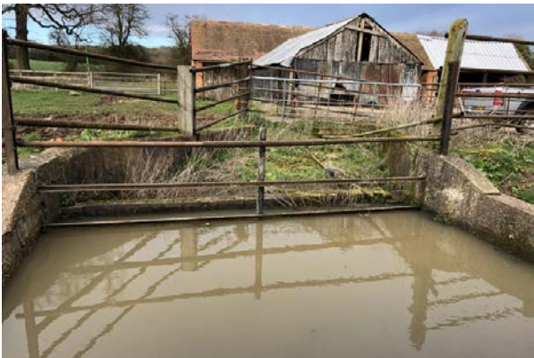
Photo showing current condition of barn
