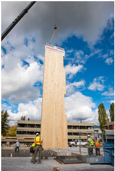
CLT lift core (SmartLam)
