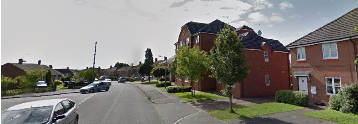
Whittington Court 3 storey flats on Whittington Drive
