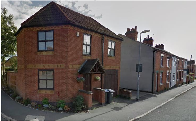
View of 100 Stamford Street (on the corner of Wolsey Drive) and 98 Stamford Street
