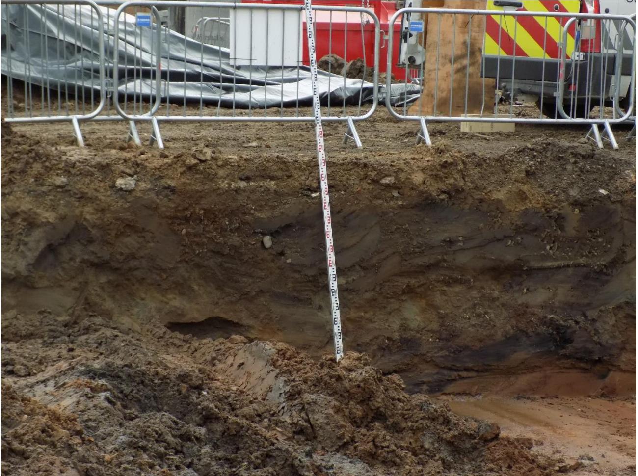
Figure 5: Photograph of Trial Pit Area
