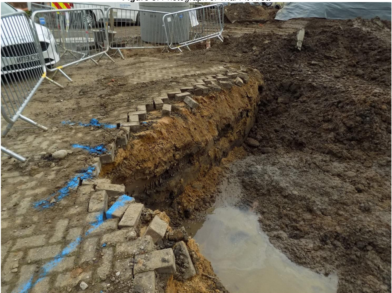
Figure 6: Photograph of Trial Pit Area
