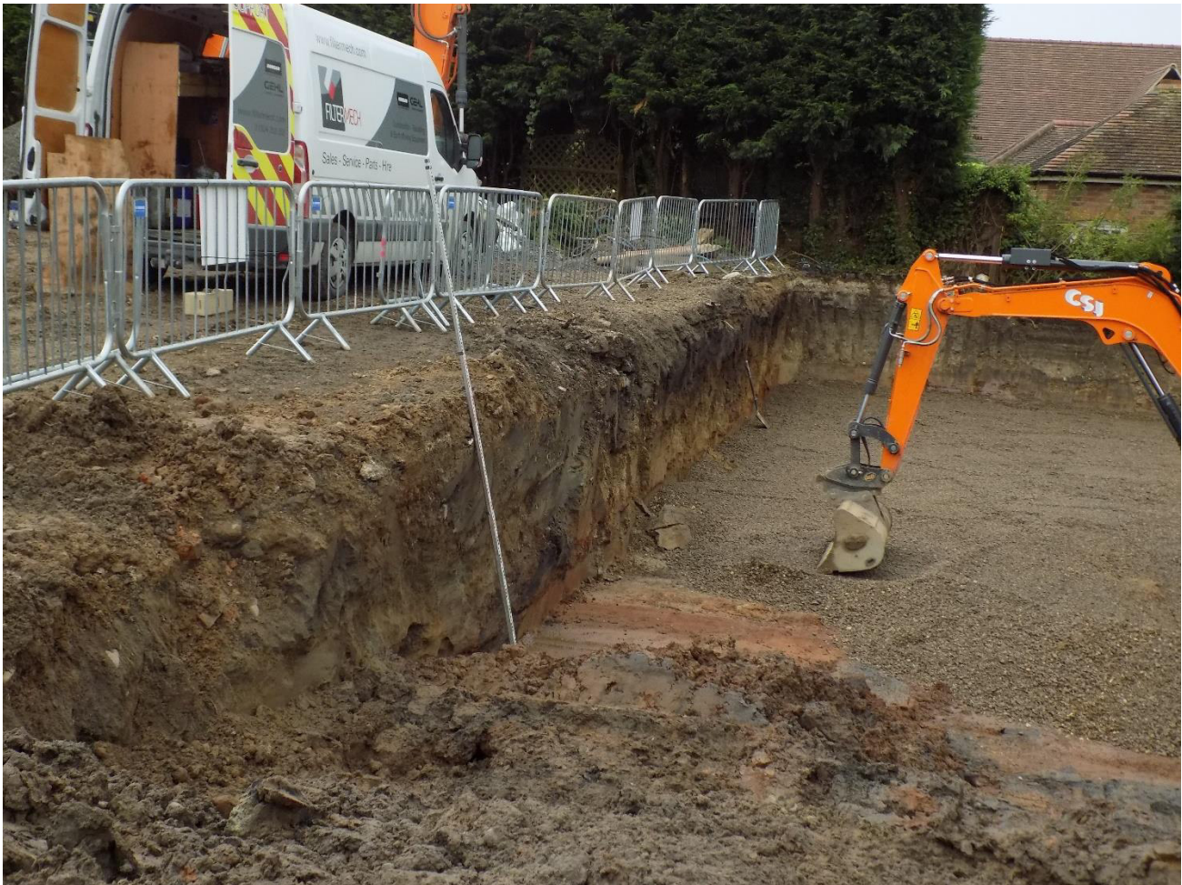
Figure 6: Photograph of Trial Pit Area
