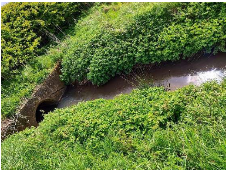
Photograph 4 – Culvert at Downstream End of Watercourse (WC2).
