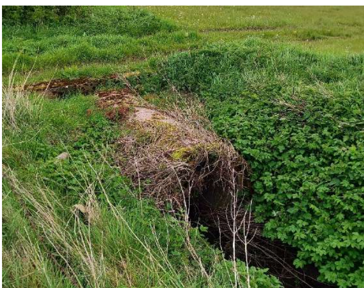
Photograph 5 – Culverted access point across WC2.
