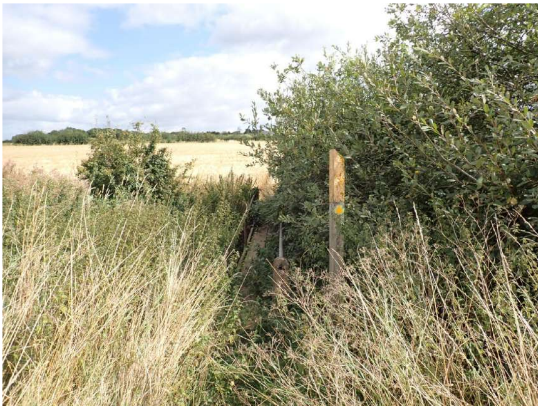
Plate 15: Footbridge across the River Mease at the north-east corner of Field 3, Site 1
