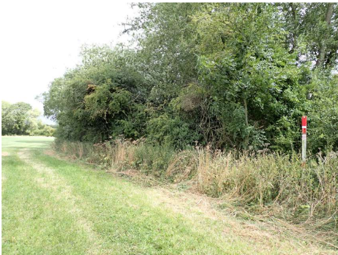
Plate 22: View of the gas pipe marker adjacent to Pessall Brook in the south corner of Field 1, Site 2
