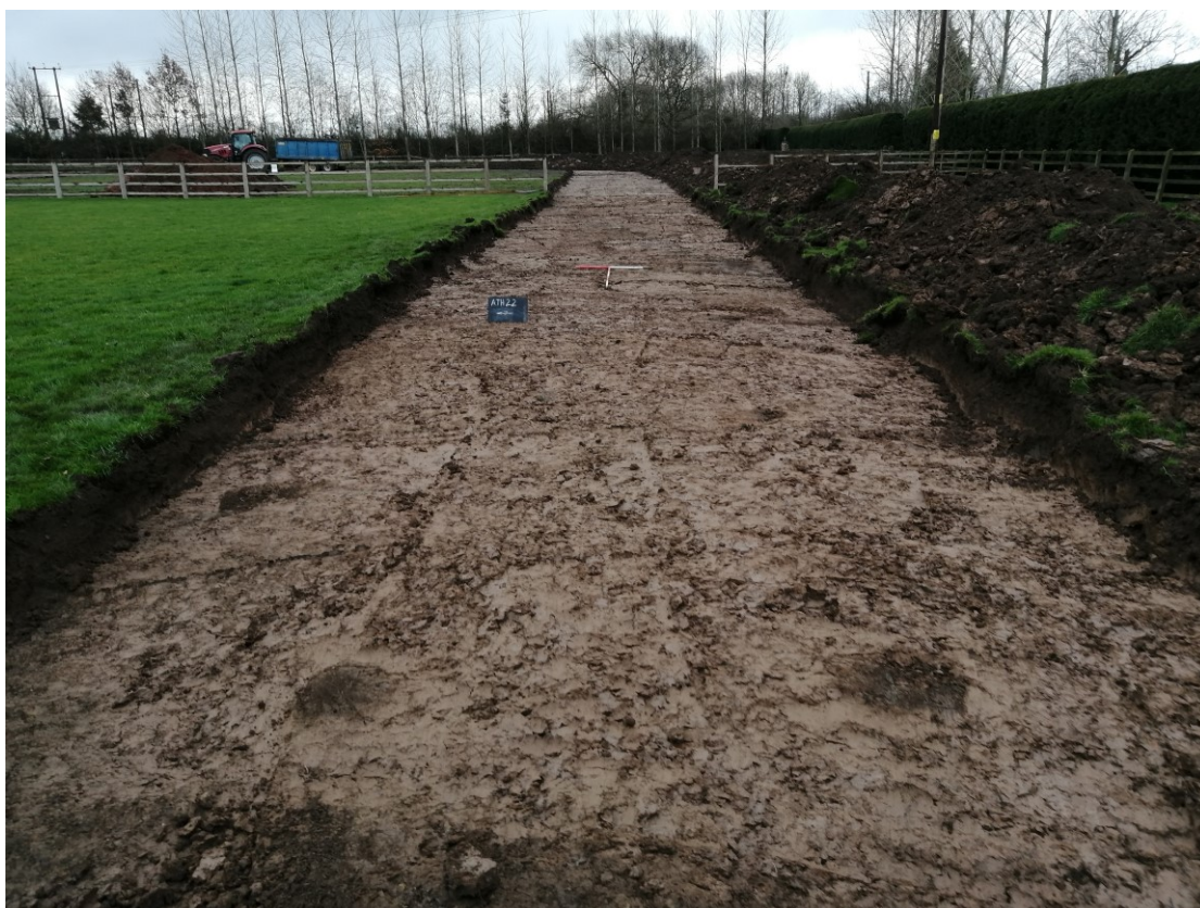
Plate 6; new access road, view east
