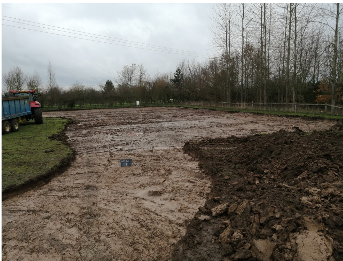
Plate 5; new access road, View northeast.
