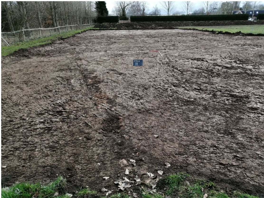
Plate 8; northern half of excavated area, view south.
