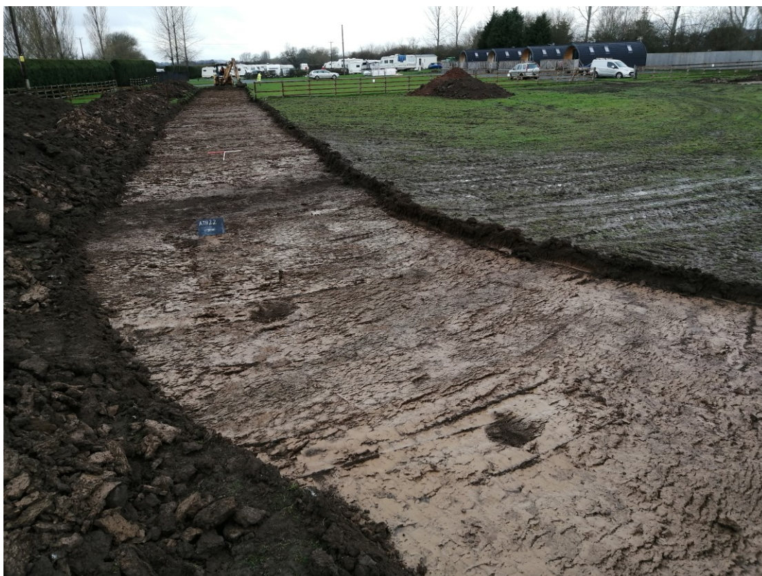
Plate 4; new access road, view east.
