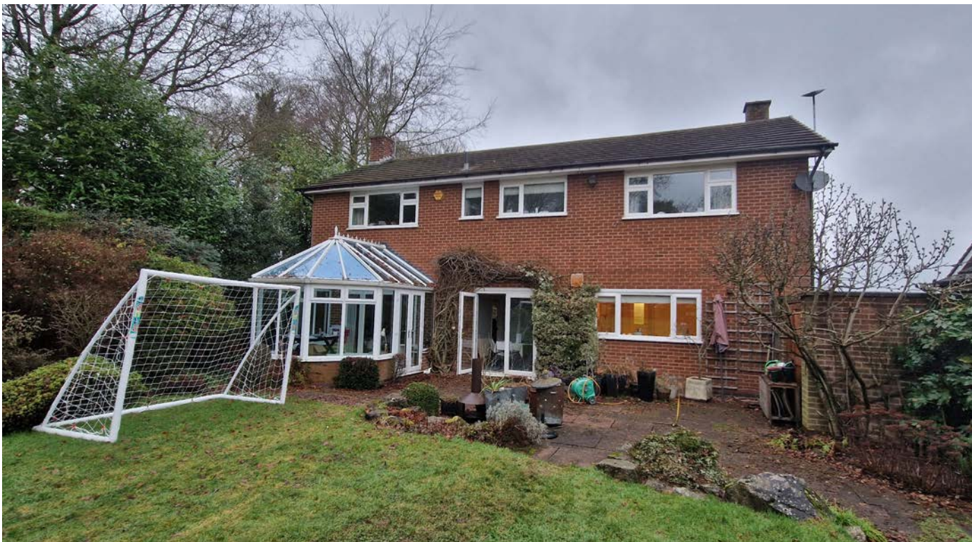
View of existing house from rear garden
