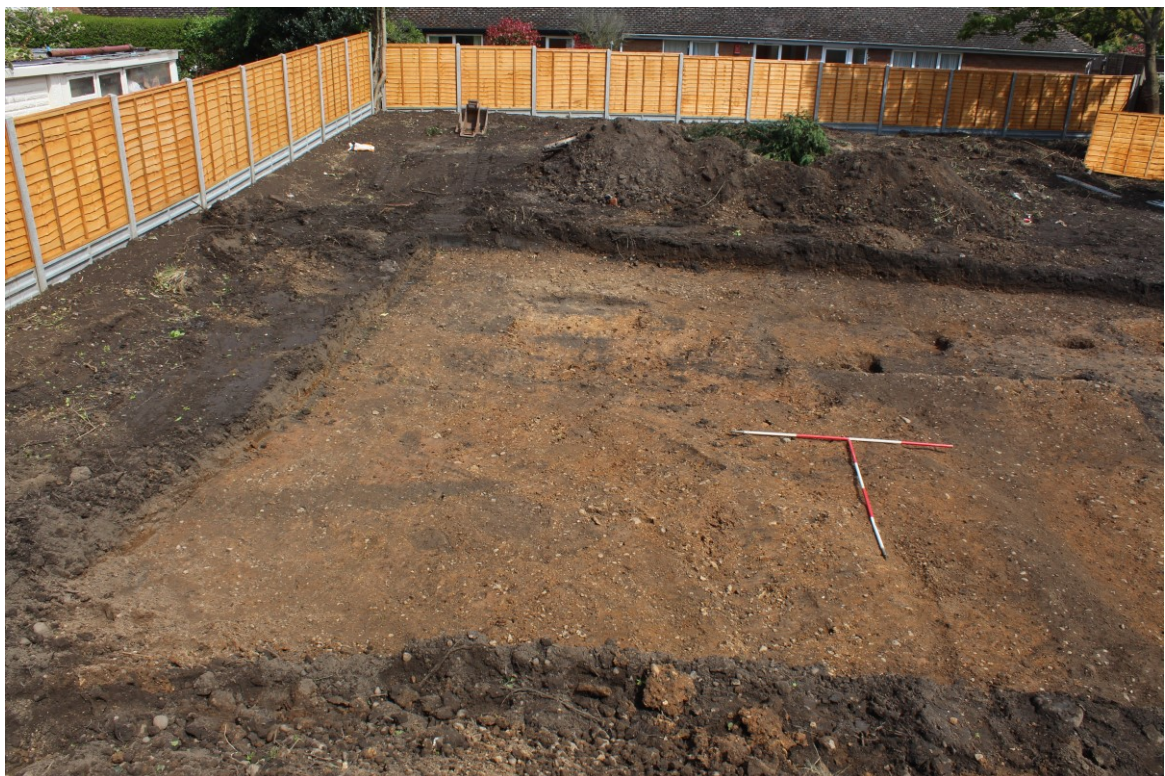
Plate 2: trench 1, north side, view east
