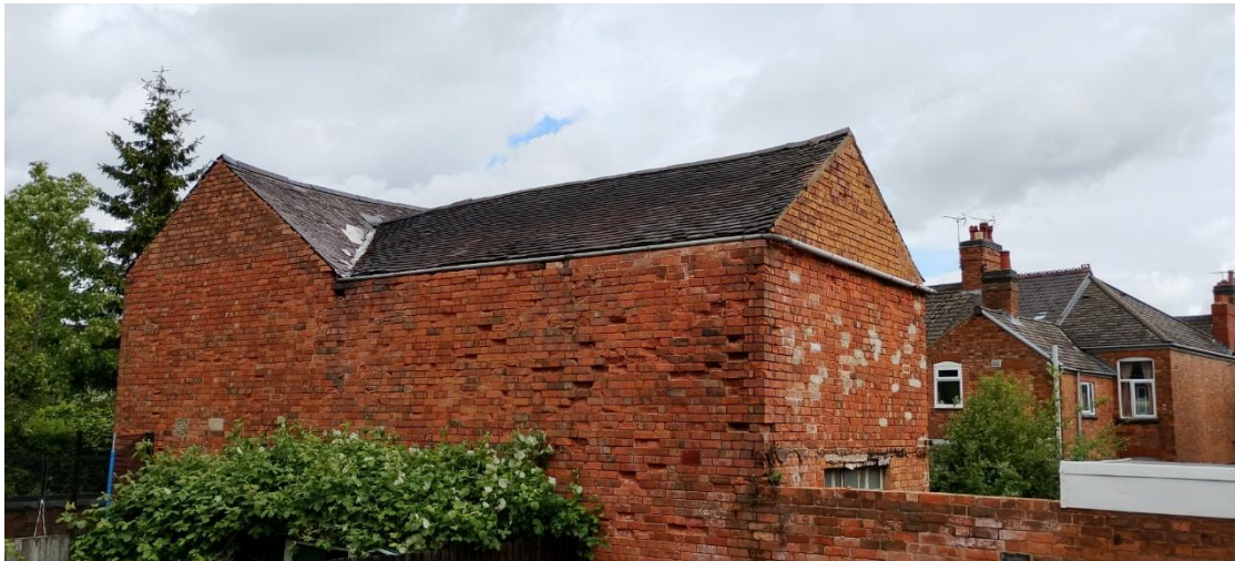
Photograph 10: External overview of surveyed building and surrounding context.
