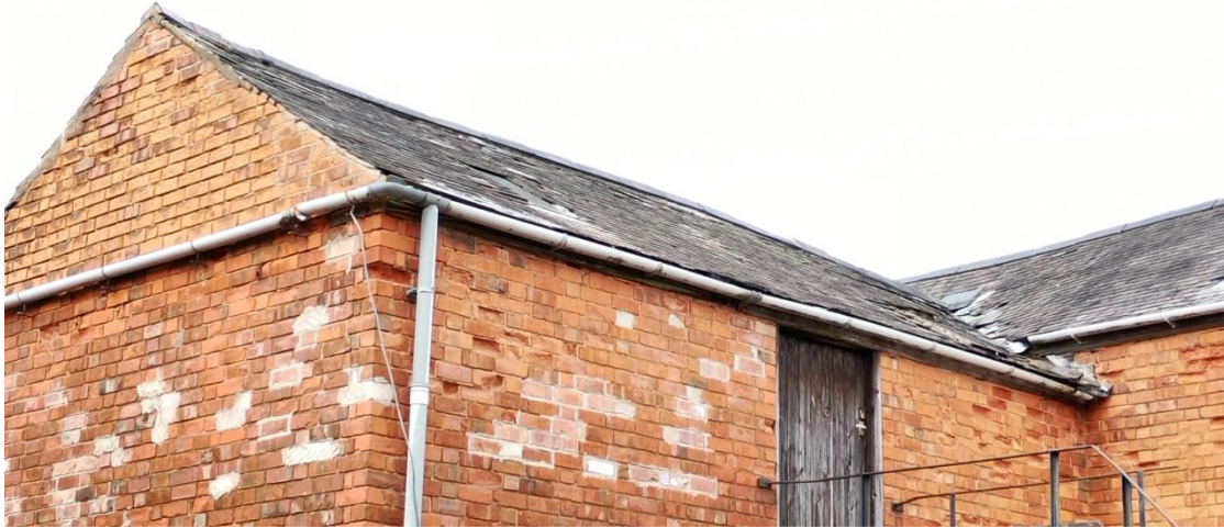
Photograph 7: External elevation showing brickwork, doorway and roof condition.
