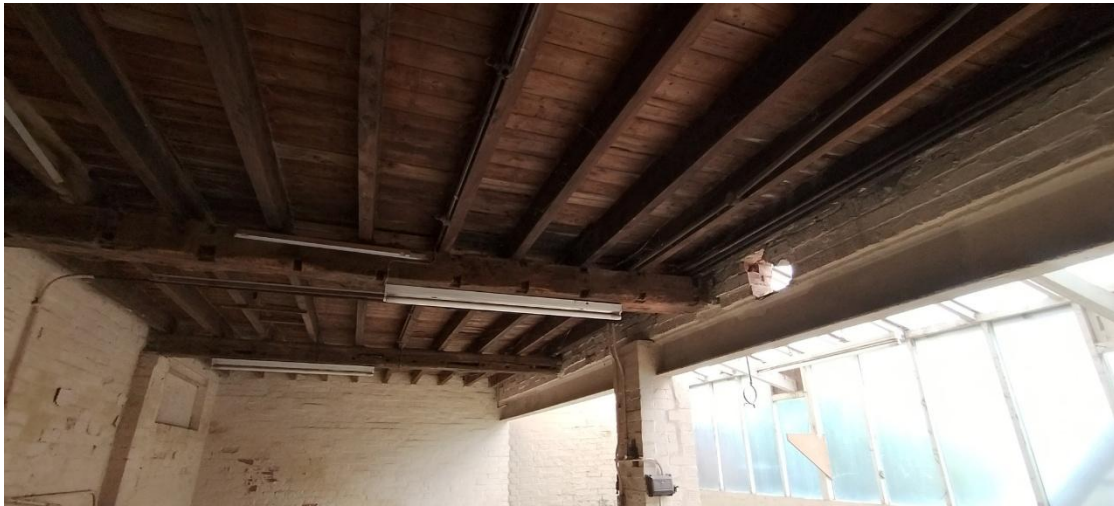
Photograph 4: Internal timber roof with exposed beams and wall opening.
