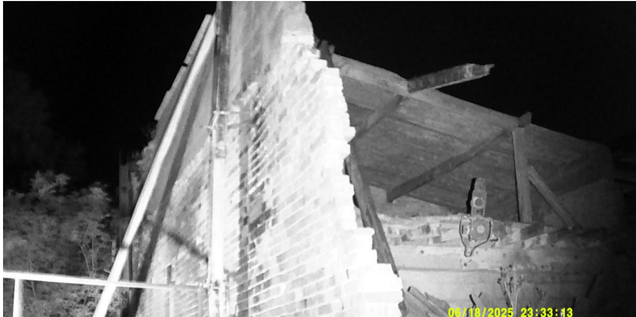
Photo 6. North and western elevations at darkest part of the survey
