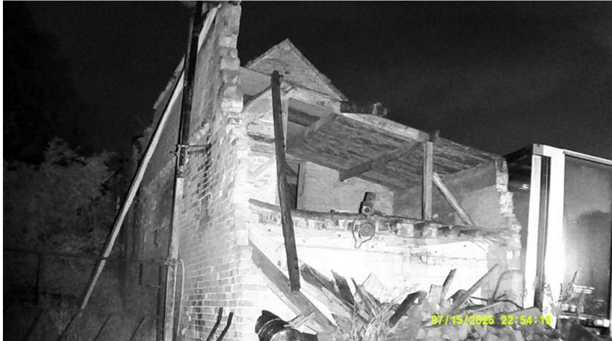
Photo 6. North and western elevations at darkest part of the survey
