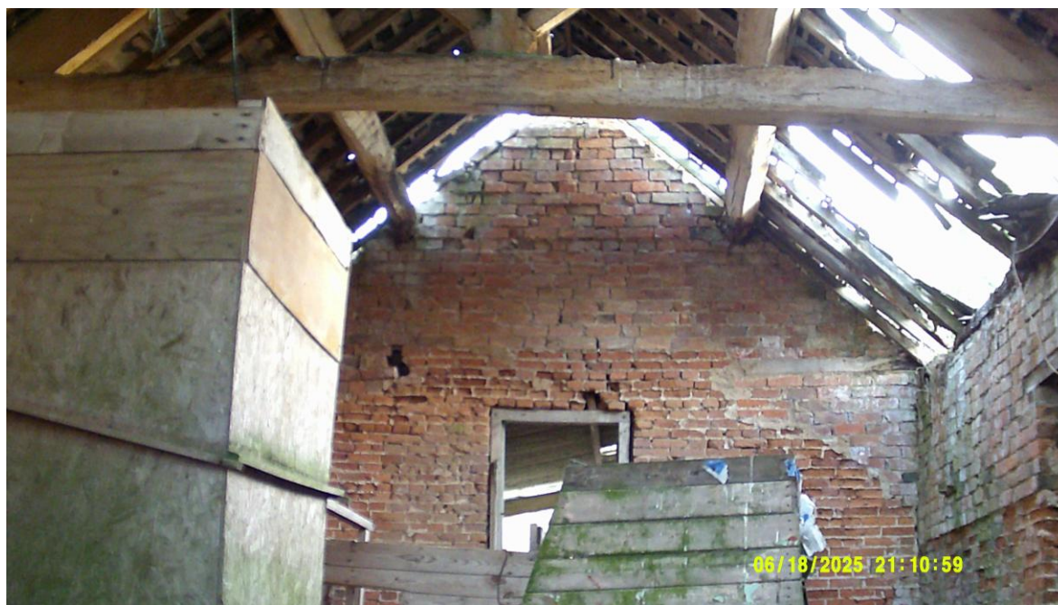
Photo 3: Internal view of the upper floor
