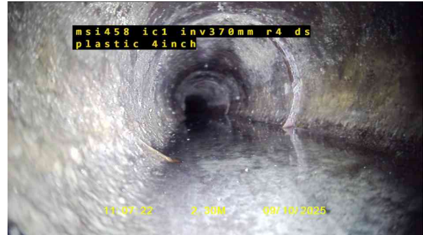
10, 00:00:44, 2.30 m Water level, 15% of the vertical dimension
