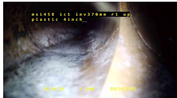
4, 00:00:19, 1.24 m Junction at 3 o'clock, 100mm dia
