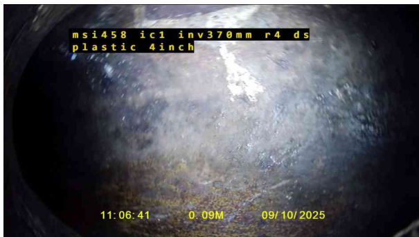
3, 00:00:04, 0.09 m Line deviates left, JOINS MAIN LINE
