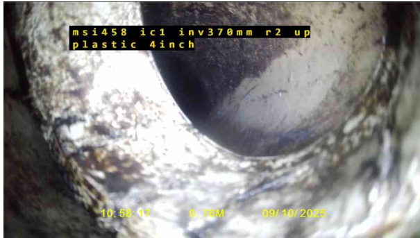
5, 00:00:25, 0.76 m General remark, PAN CONNECTOR IN LINE
