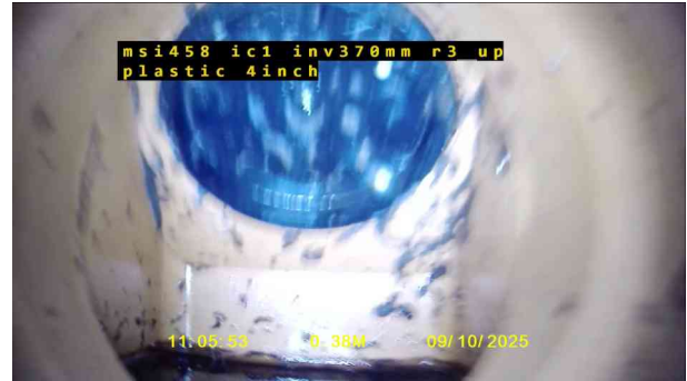
2, 00:00:05, 0.38 m Finish node, gully, reference: R3
