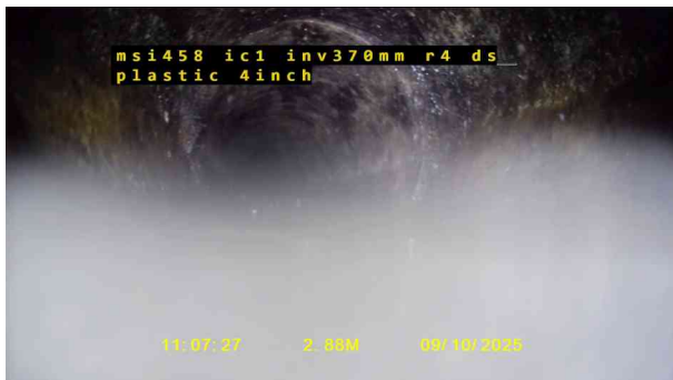
11, 00:00:49, 2.88 m Loss of vision, camera under water, start
