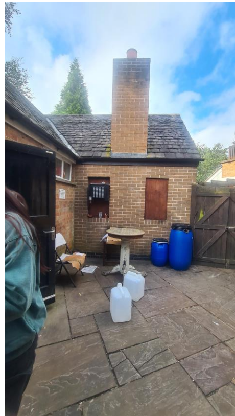
Image B: The existing Storage space
