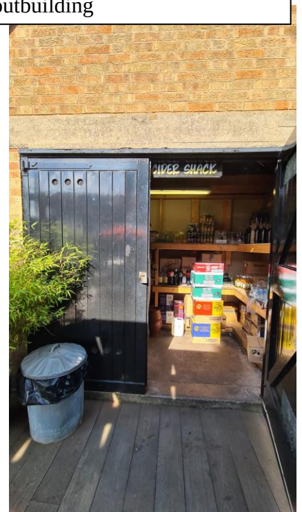
Image D: The existing Storage outbuilding
