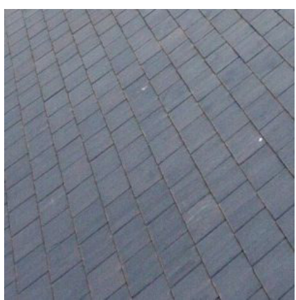
ROOF TILES: Natural Slate to main roof and porches.
