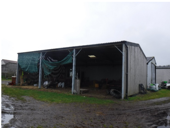
Photo 1. Section B1b – external, eastern elevation.
