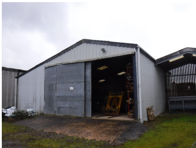
Photo 2. Section B1a – external, northern elevation.
