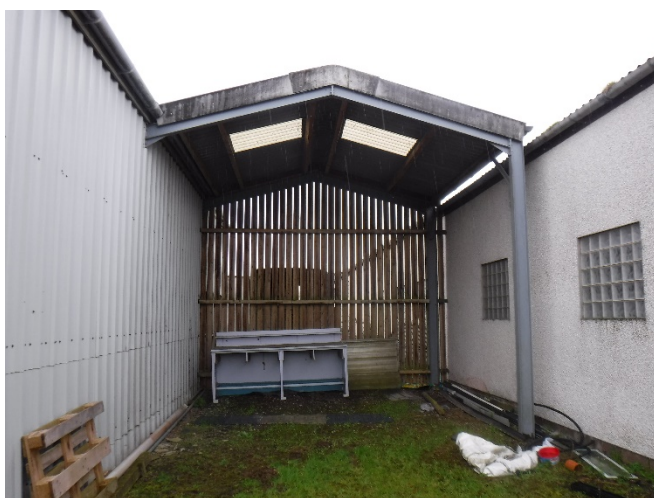
Photo 3. Section B1c – northern elevation.
