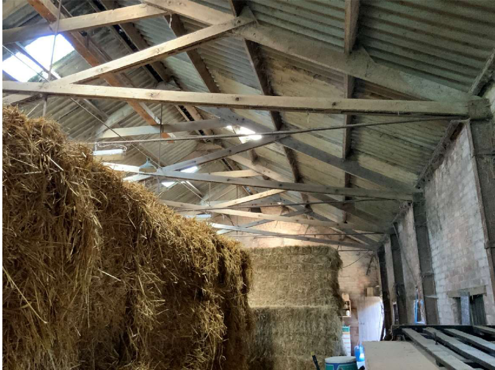
Picture 31 – further view of roof trusses and tie bars of lower member
