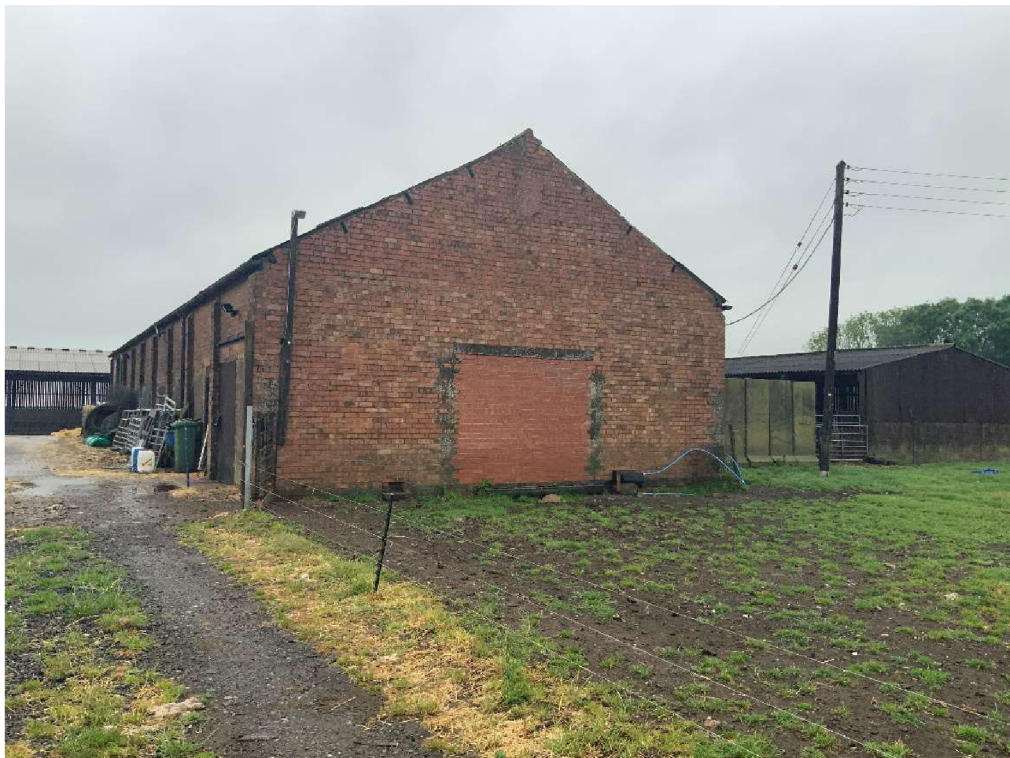
Picture 42 – North gable view 2023
