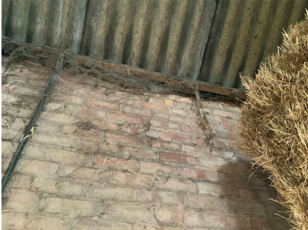
Picture 41 – Purlin adjacent to eaves walls in good condition
