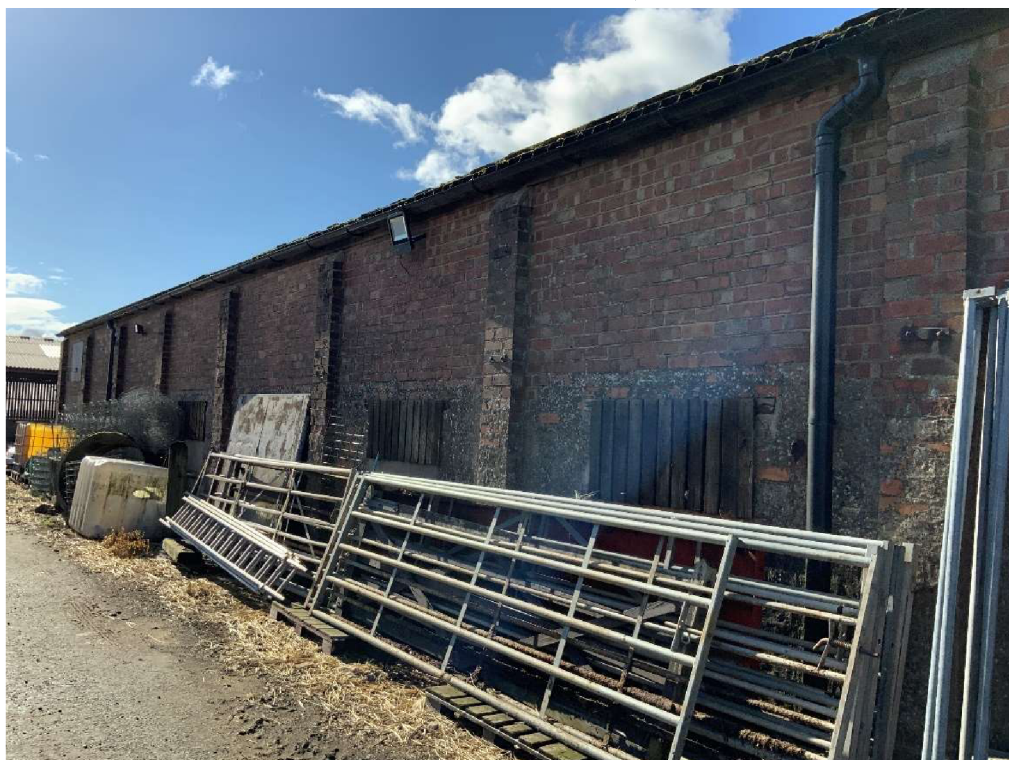
Picture 4 – General eastern elevation showing render line
