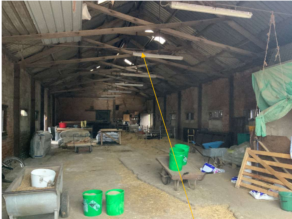
Picture 45 – Cleared interior of barn 2023 – note minor bend in tie bar of truss
