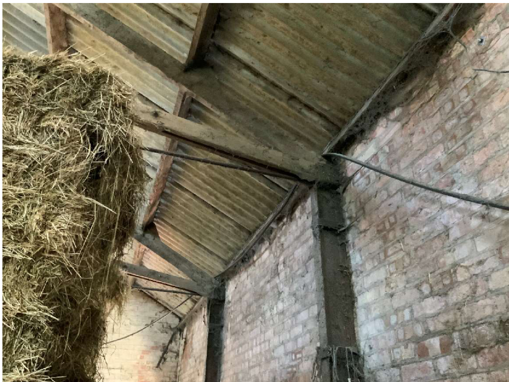
Picture 36 – closer detail of connection
