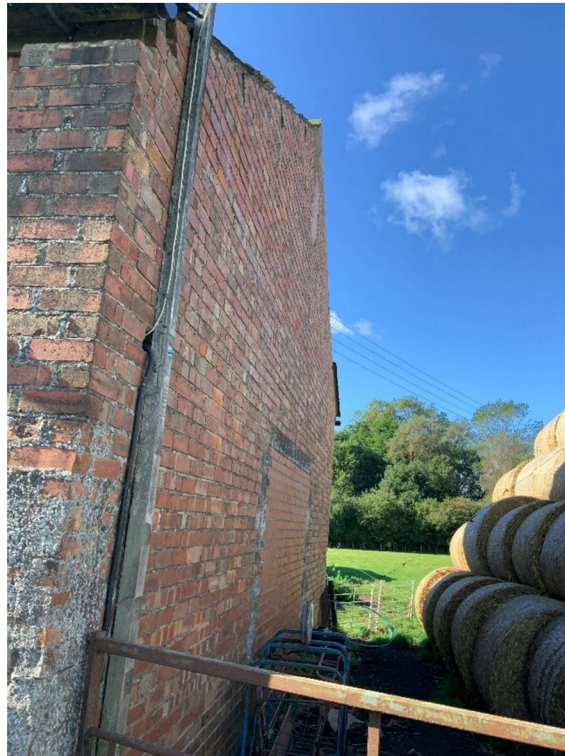
Picture 1 – North end gable infilled doorway and exposed verge
