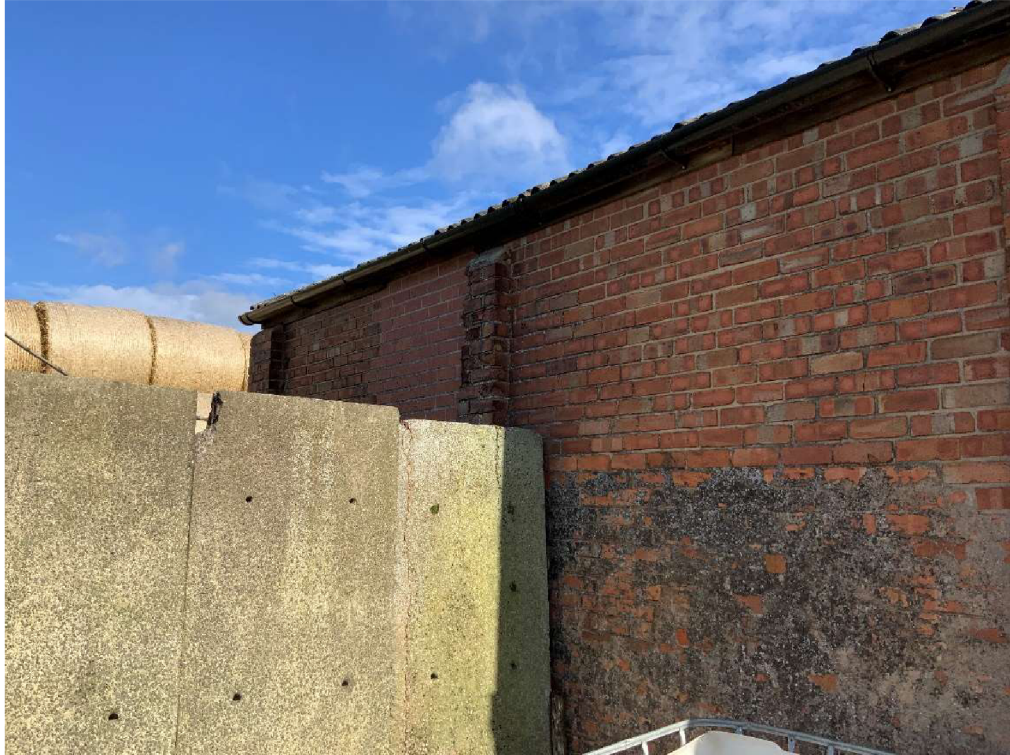
Picture 19 – replaced brick panel behind retaining wall panel
