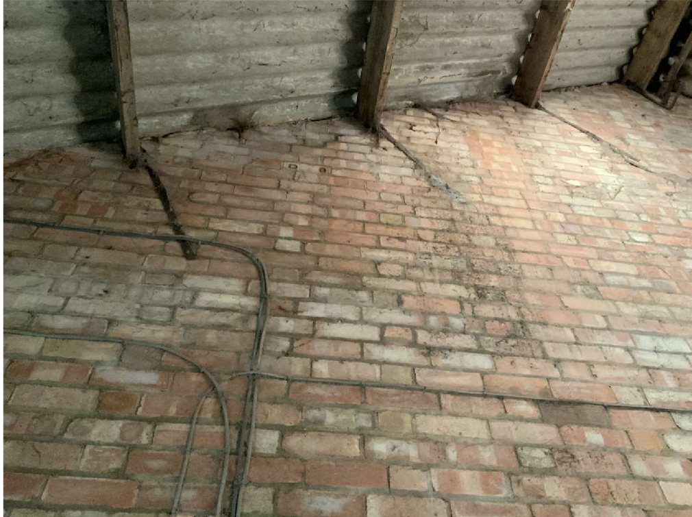
Picture 25 – Purlin holding down straps adequate
