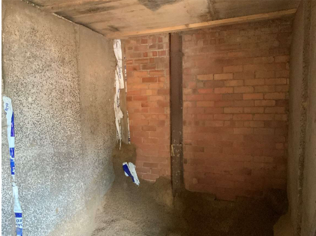
Picture 29 – Internal partition to south eastern corner
