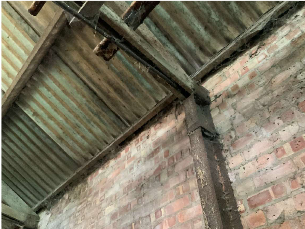
Picture 35 – Truss/Column connection
