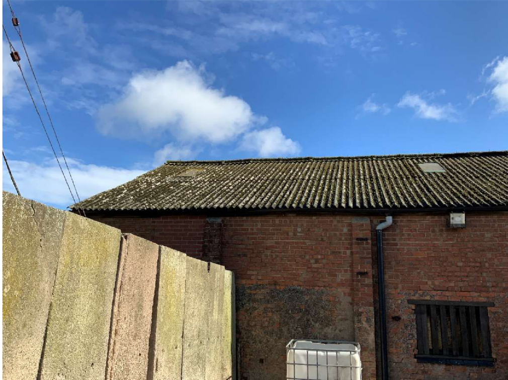
Picture 21 – General roof line good
