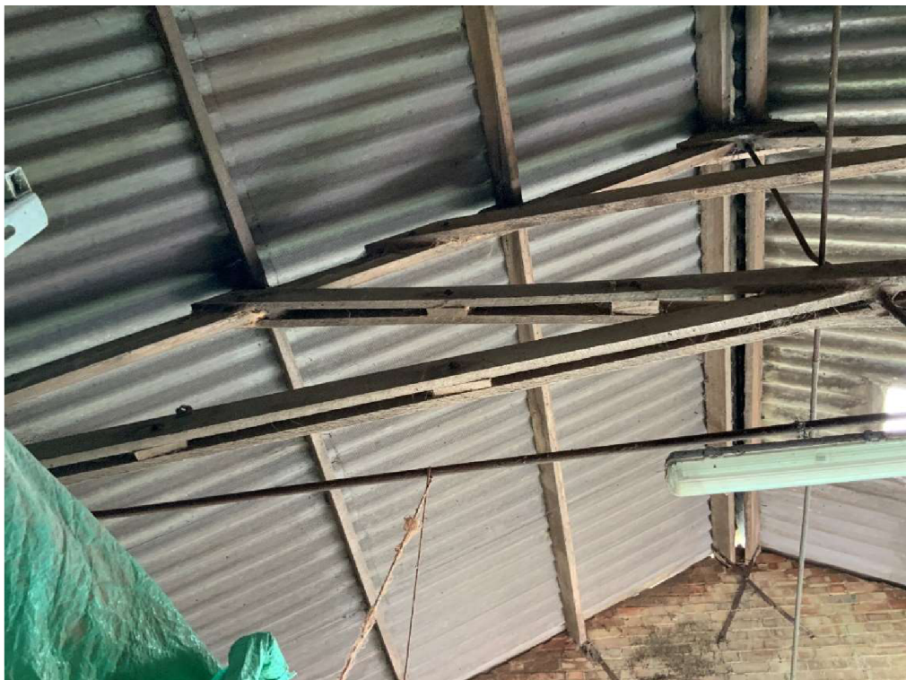
Picture 38 – truss connection details
