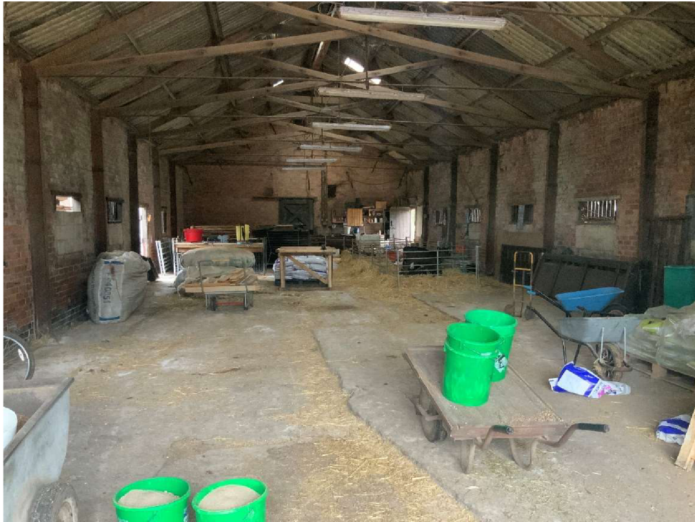
Picture 47 – Interior of cleared barn 2023 - note floor level difference to centre
