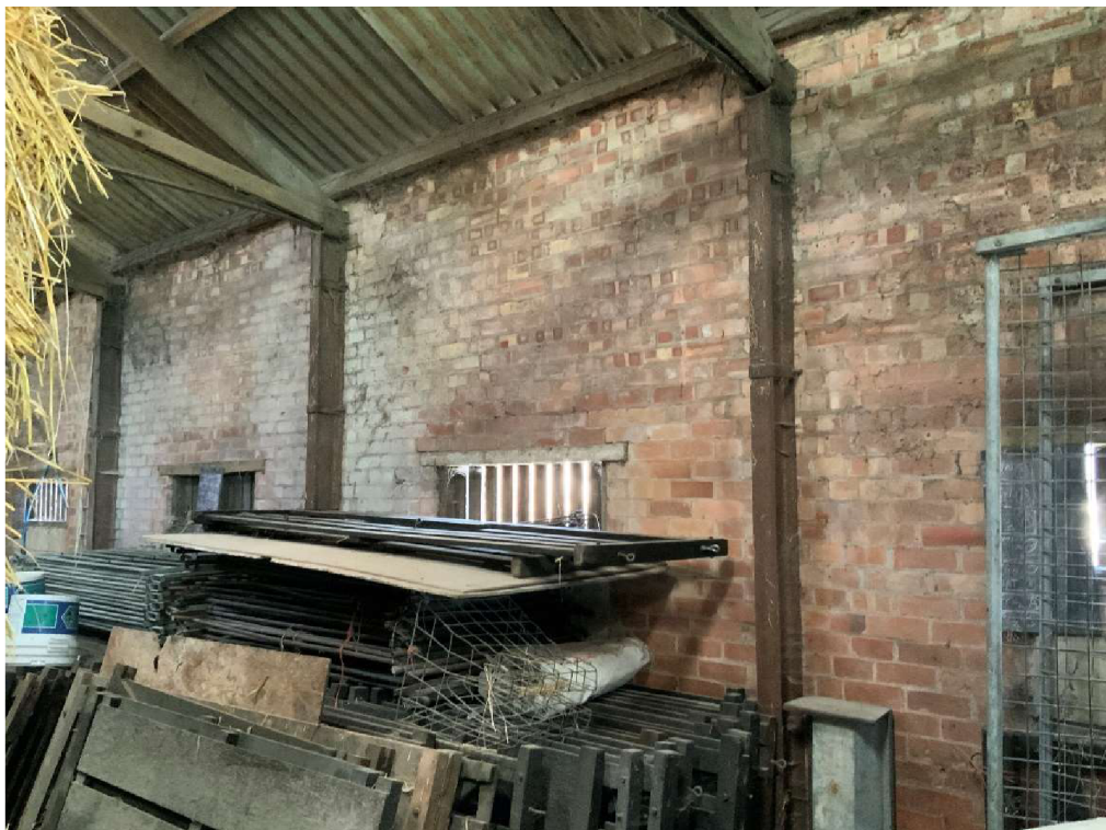
Picture 30 – detail of columns and timber trusses to roof
