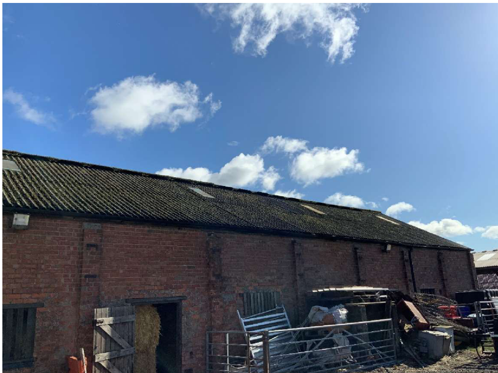
Picture 22 – General roof line good ACM roof panels will need replacement
