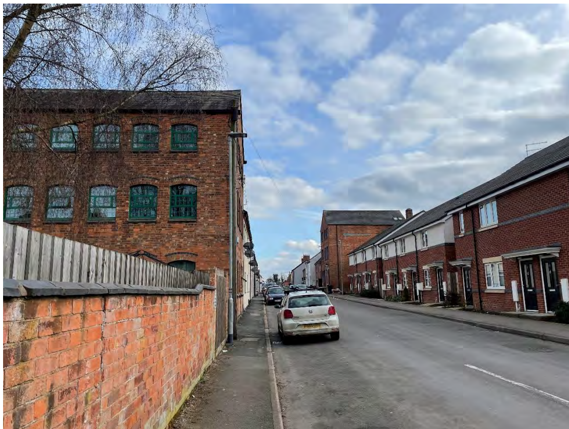
Graphic 9.4 Key view in Earl Shilton Conservation Area towards 1-5 New Street (formerly A Abbott Ltd)
