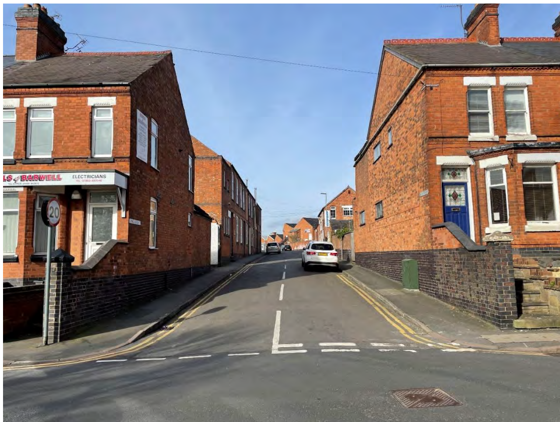
Graphic 9.2 Key view in Barwell Conservation Area
