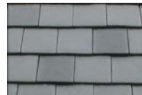
Grey interlocked roof tiles
