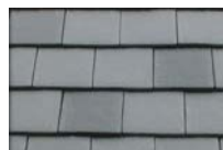
Grey interlocked roof tiles
