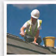
Nearly 200 construction jobs could be provided directly on site
