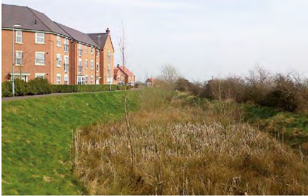
Established sustainable drainage features on adjacent site
