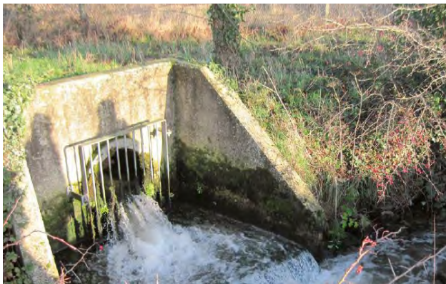
Outfall from WWTW
