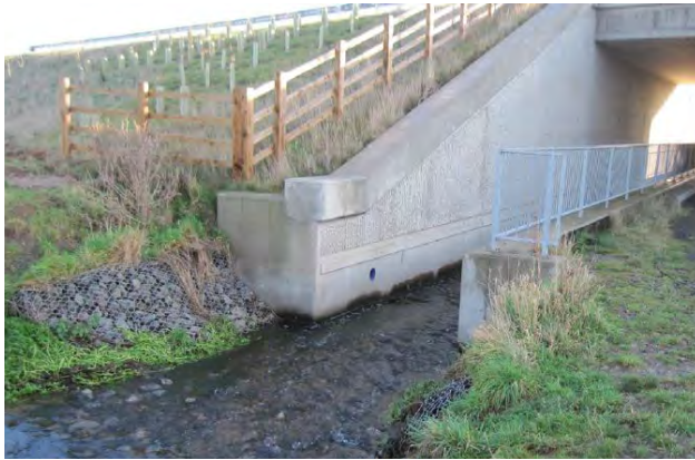
Earl Shilton Brook at underpass beneath A47
