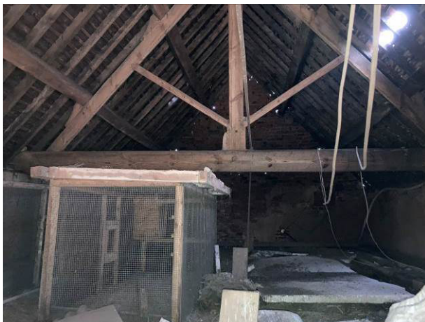
Roof space interior east side
