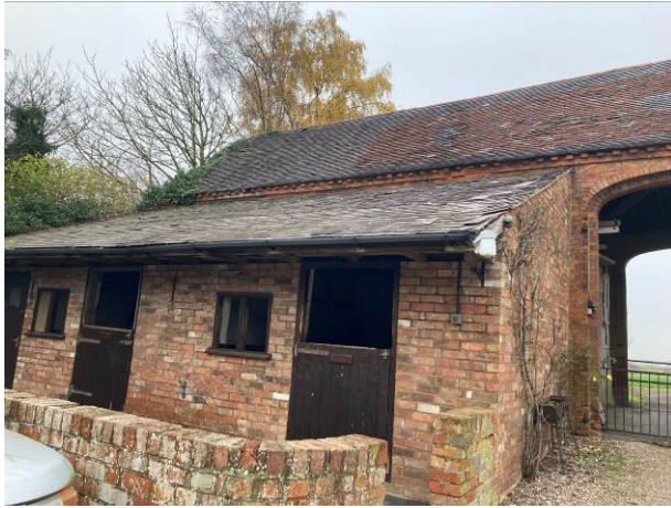
South west side B3 and B4
