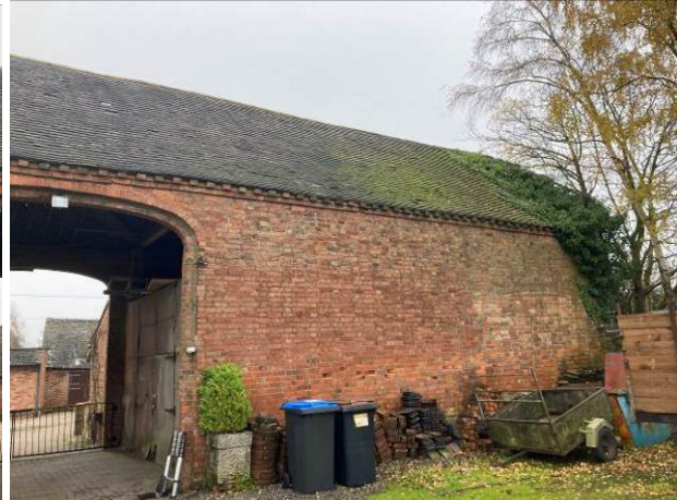
North west side B3
