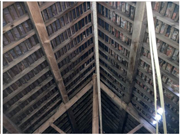
Underside of roof west side
