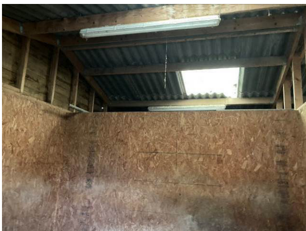
Interior of B6
