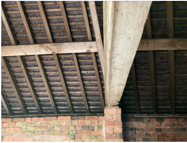
Underside of roof east side
