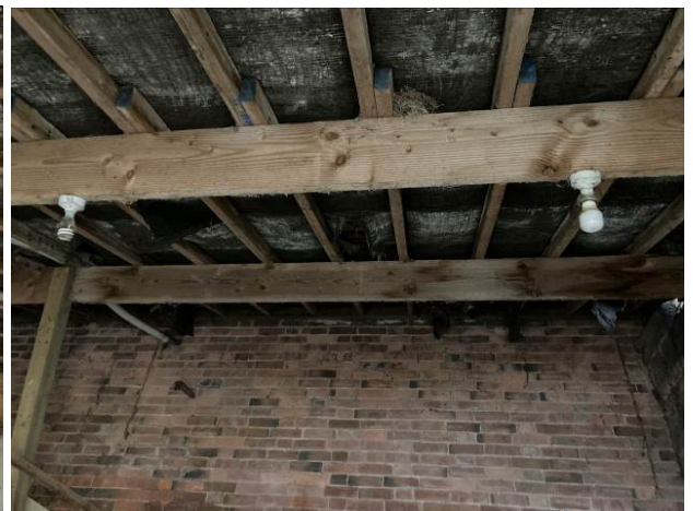
Interior of B4 lean to extension
