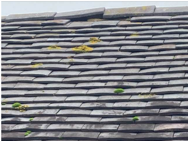
Close up of tiled roof B2
