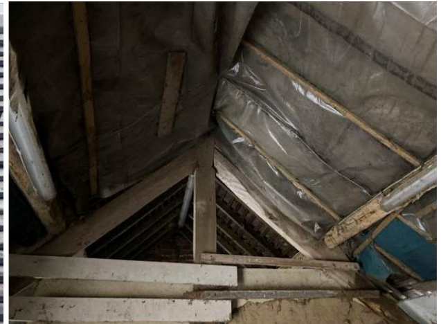
Open underside of roof B2
