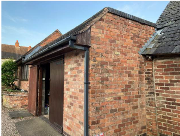
North face of garage
