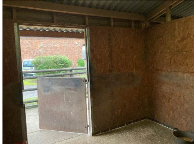
Interior of B5
