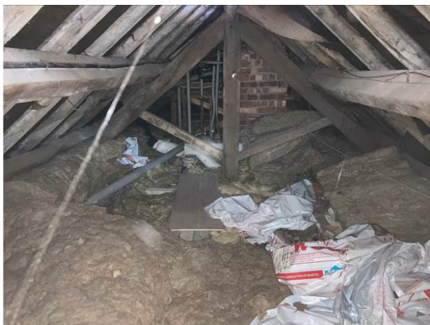
Bungalow loft interior
