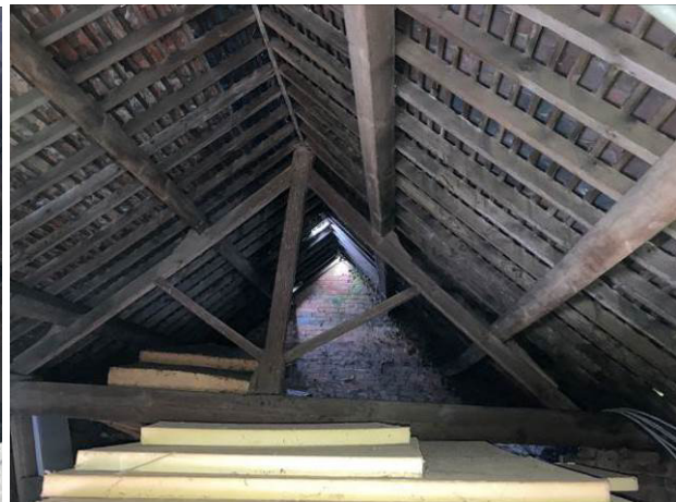
Roof space interior west side
