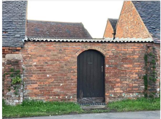
South face of garage
