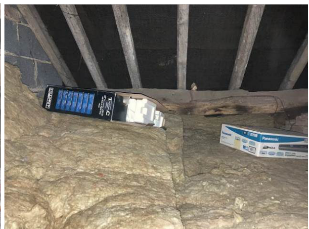
Bungalow loft interior
