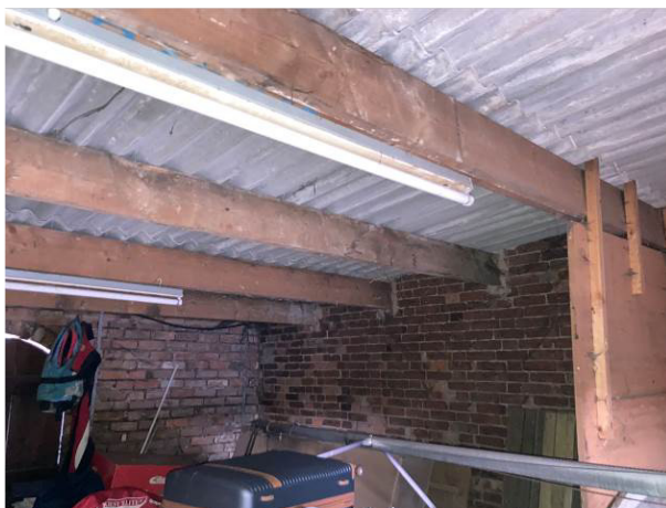
Interior roof of garage
