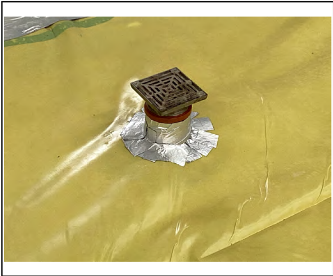
View of a typically sealed pipe
