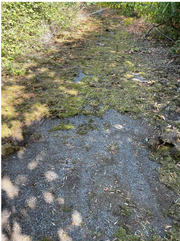
Figure 1.6 - Existing asphalt visible on Wolvey Road
