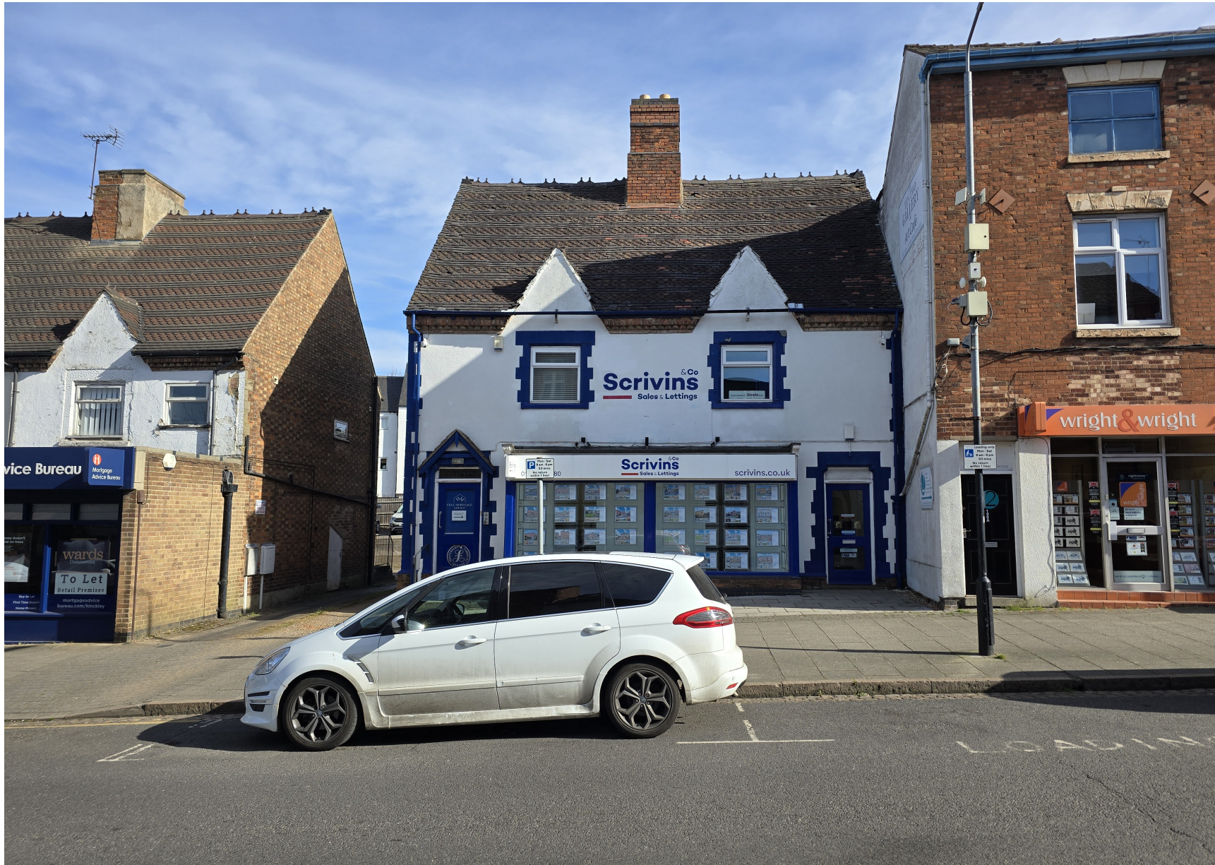
The front of 96-98 Castle Street, as seen from the road. Image credit: M. Gatehouse (April 2025).
