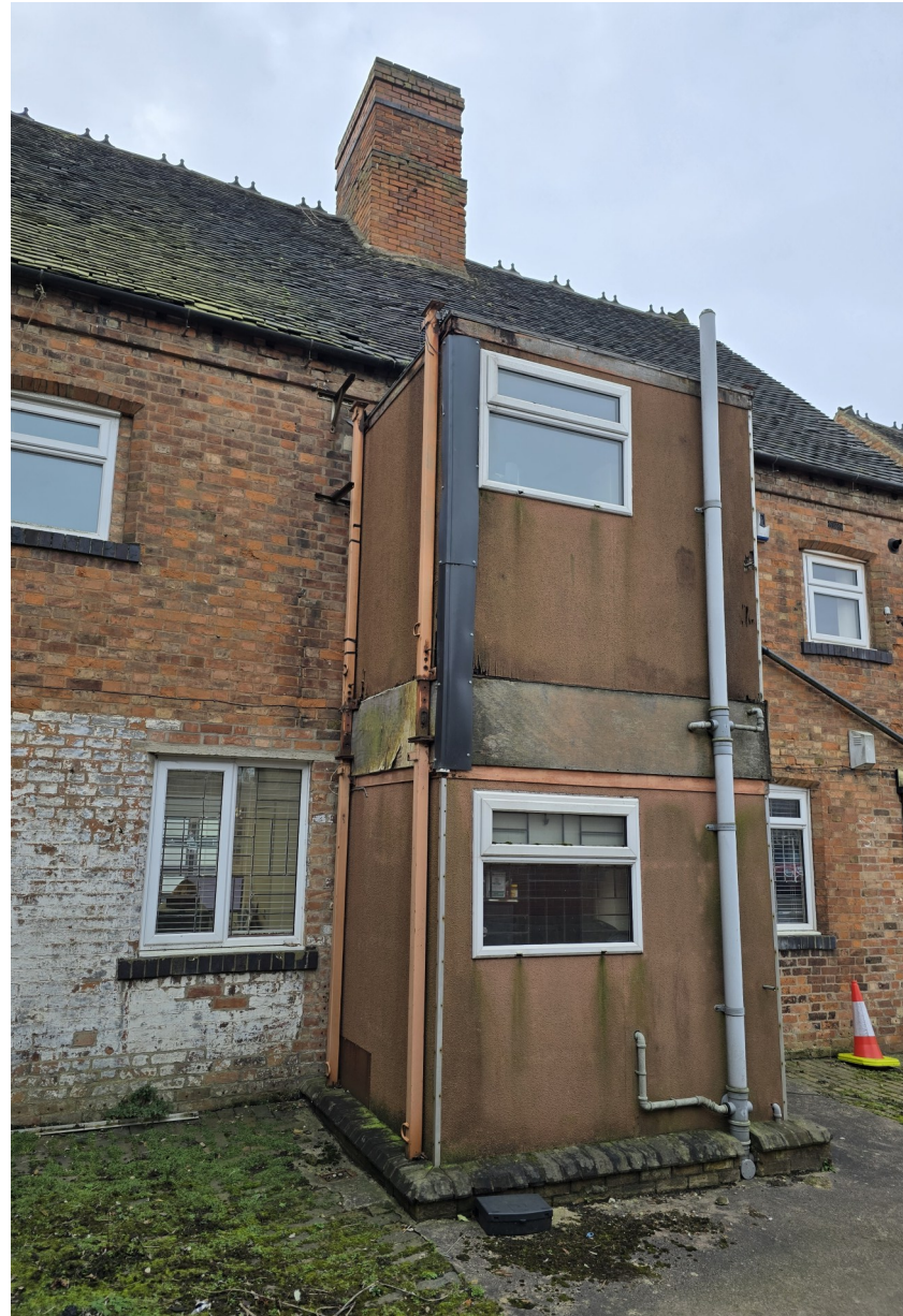
Two views of the rear of 96-98 Castle Street, showing the existing extension. The form and massing of the existing extension is not in keeping with the original building, and represents an inappropriate addition given the historical context of the site. Image credits: M. Gatehouse (February 2025).
