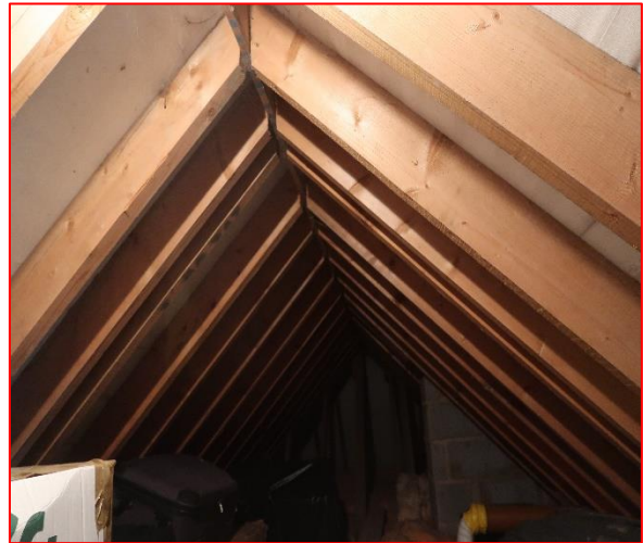
Internal view of roof space
