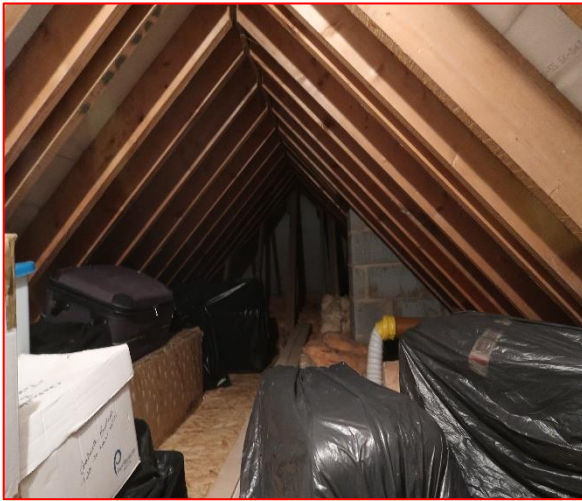
Internal view of roof space
