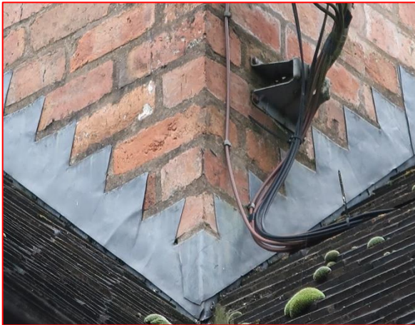
View of chimney and lead flashing
