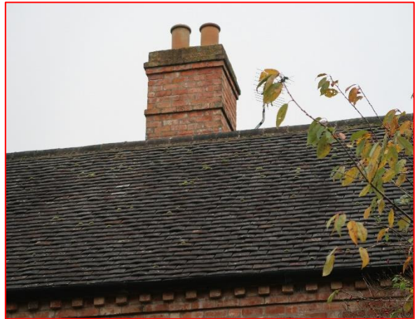
View of roof
