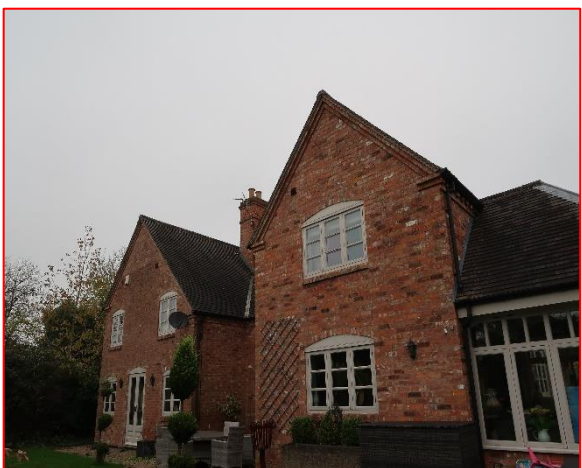
View of gable end – location of extension
