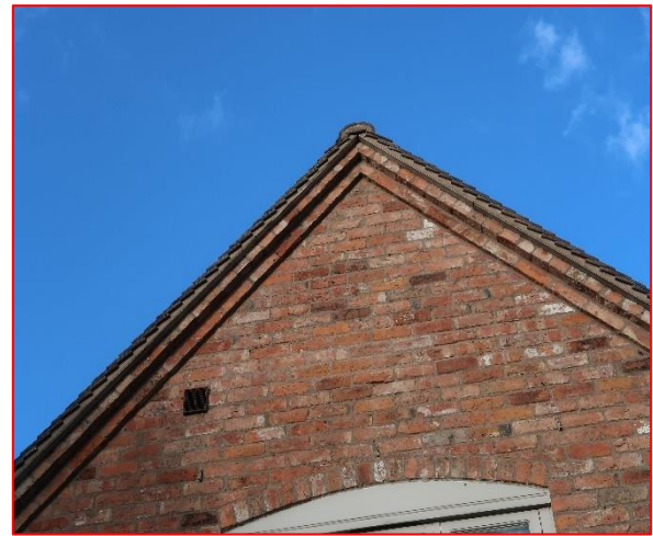
View of gable end
