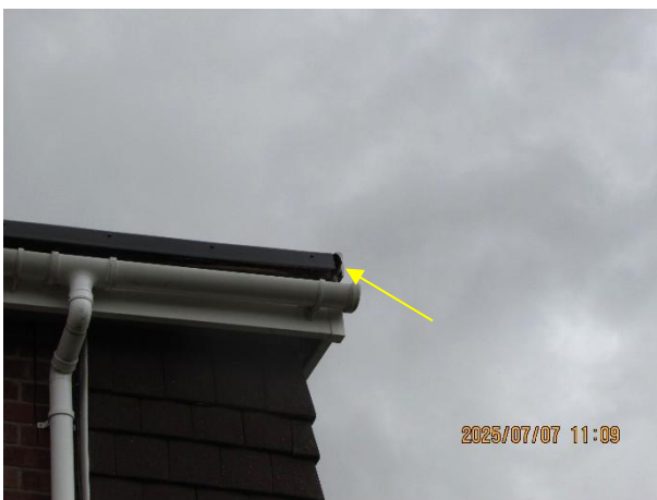
Gap at corner of flat roof
