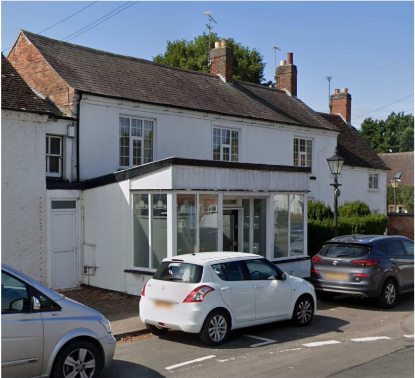
Street view of 18, 20 and 20A, Main Street
