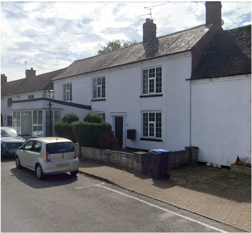
Street view of 18, 20 and 20A, Main Street
