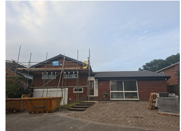
Figure 1a: The front side of B1, with scaffolding present on the left side.
