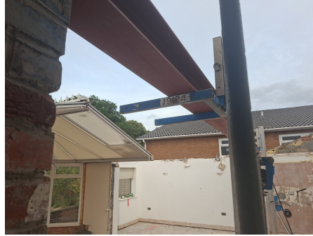
The removed roof of B1 (removed on the right/ Eastern side).
