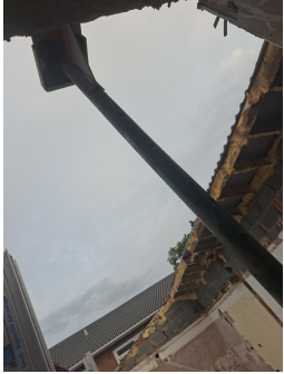
The removed roof of B1 (removed on the right/ Eastern side).
