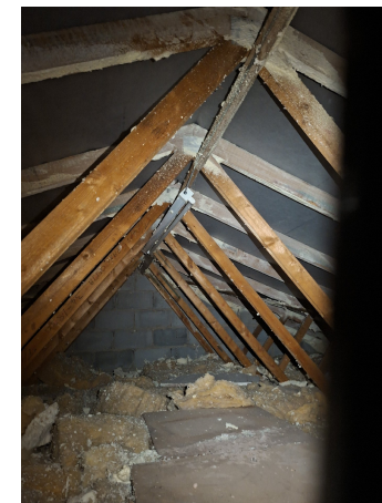
Figure 1b: The internal loft space of B1, on the left side of the building. The internal void is largely the same apart from the lack of foam insulation previously present on the roof. The roof itself was also retiled.
