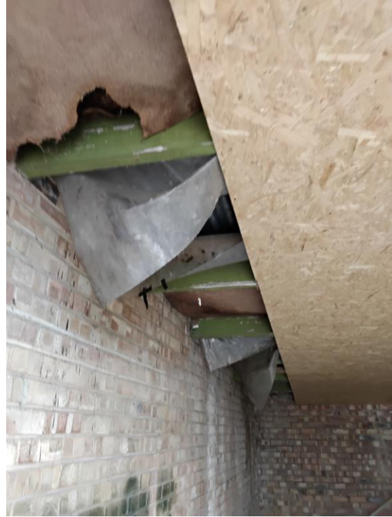
Left: Photo 3 – Roof void of the main garage. The roof was lined with MDF boarding, with evidence of damp throughout.
