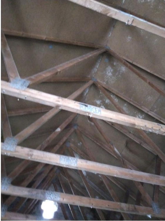
Left: Photo 3 – Roof void of the main garage. The roof was lined with MDF boarding, with evidence of damp throughout.
