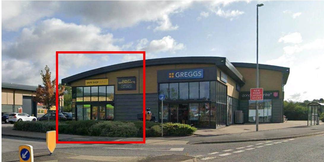
Photo 1: West elevation of application site
