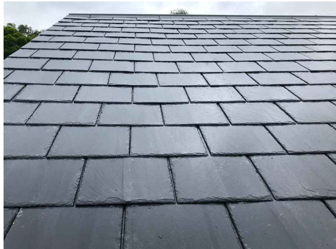
Example Roof Covering
