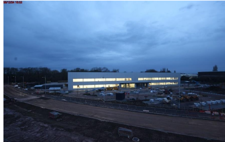
Photo 14: Internal fitout complete
