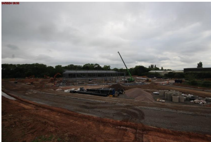
Photo 7: Continued steel frame and ground levelling progress
