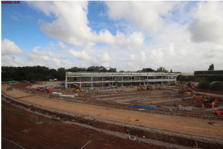
Photo 9: Completed steel frame
