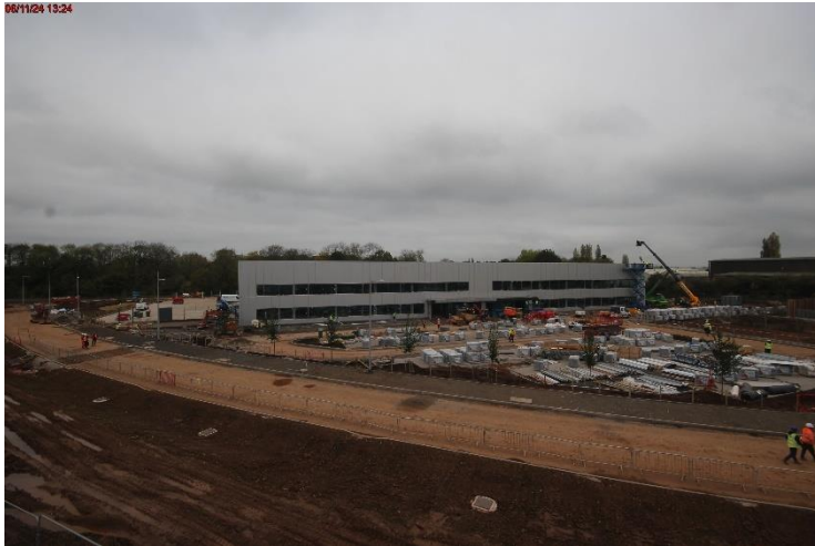
Photo 13: External façade complete, Internal fitout in progress
