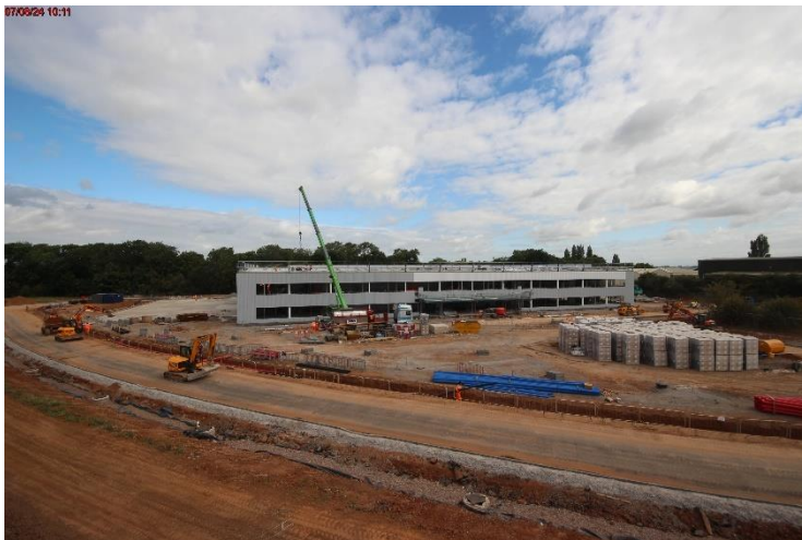
Photo 11: External façade progress
