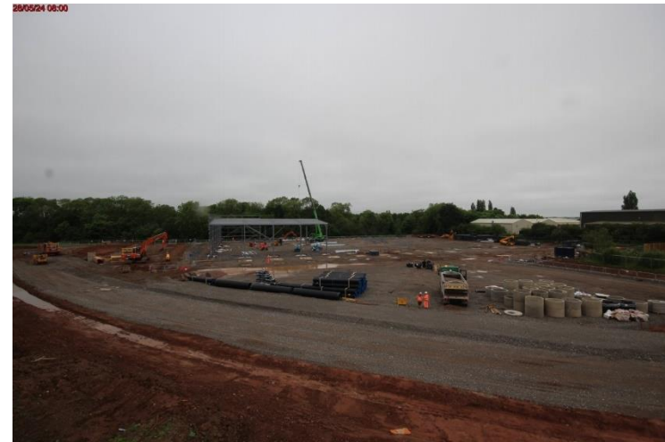
Photo 6: Steel frame construction commencement
