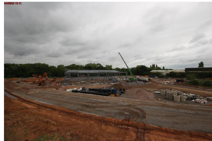
Photo 8: Continued steel frame and ground levelling progress
