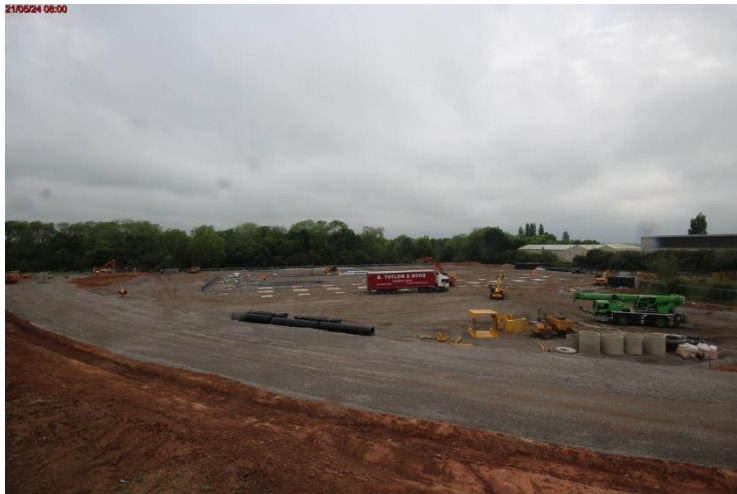
Photo 5: Ground buildup ongoing
