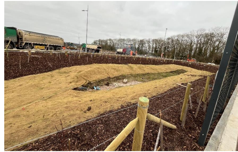
Photo 16: Temporary surface drainage point
