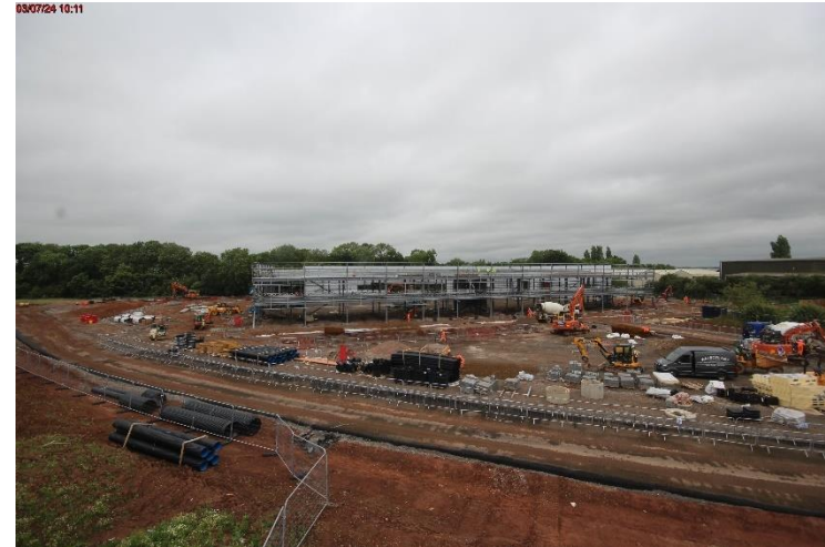
Photo 10: External façade works
