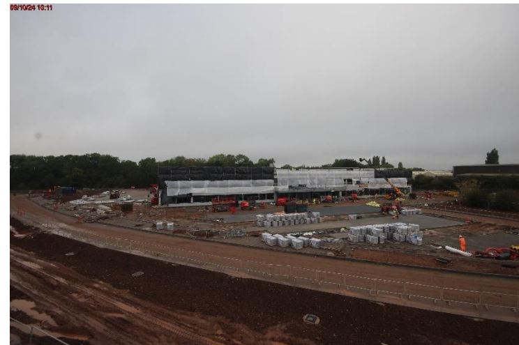
Photo 12: Ongoing external façade and internal fitout progress
