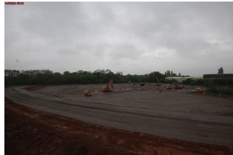
Photo 4: Ongoing Type 1 crush placement
