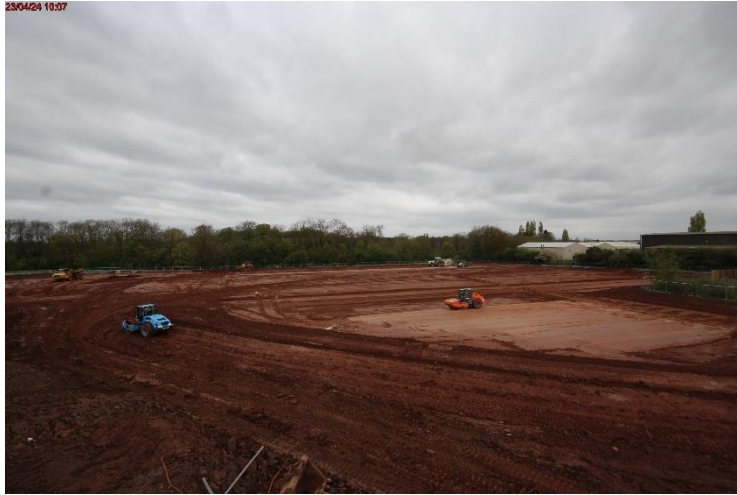
Photo 1: Initial ground stabilisation and preparation
