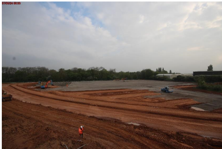
Photo 3: Type 1 crush placement for site releveling
