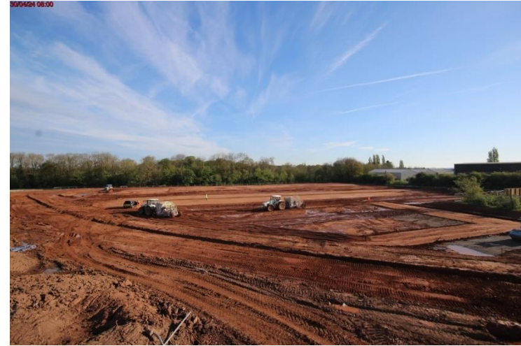
Photo 2: Ongoing ground stabilisation works
