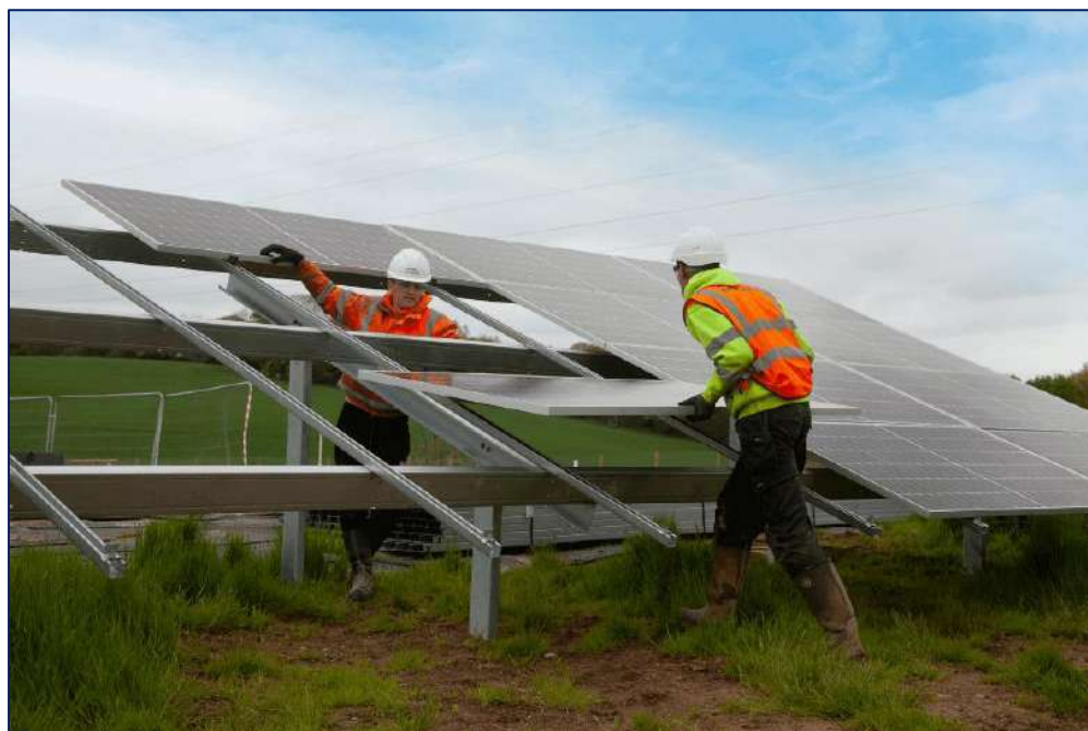
Plate 4: PV module installation 2
