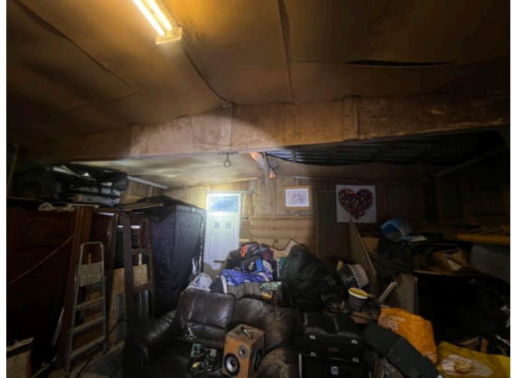
Photo 6: Existing building interior
