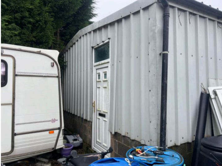
Photo 5: Existing building exterior
