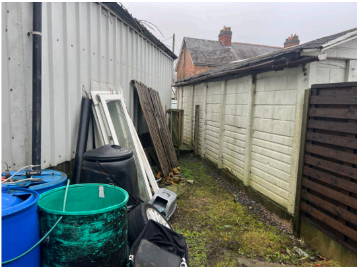
Photo 3: Side of property and existing garage (left)
