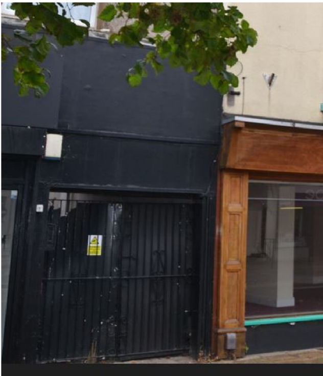
Fig. 4 Access gates to Slaughter House Yard
